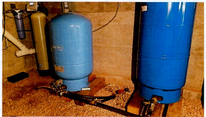
pressure tank installation
