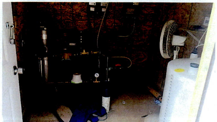
Pump house appurtenances
