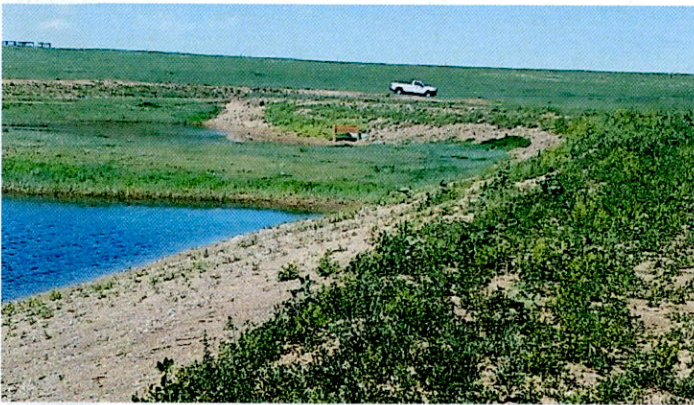
Top of embankment and front slope from east end of fill
