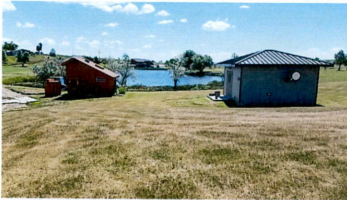
Pond pump site to left, booster for city supply right
