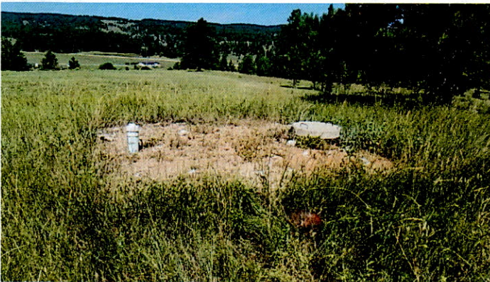
Well cap (lower right foreground), 5,000 gallon cistern (center)
