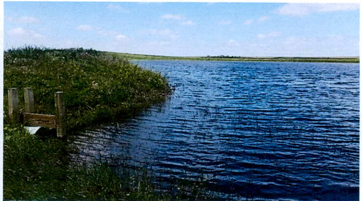
Principal Spillway inlet
