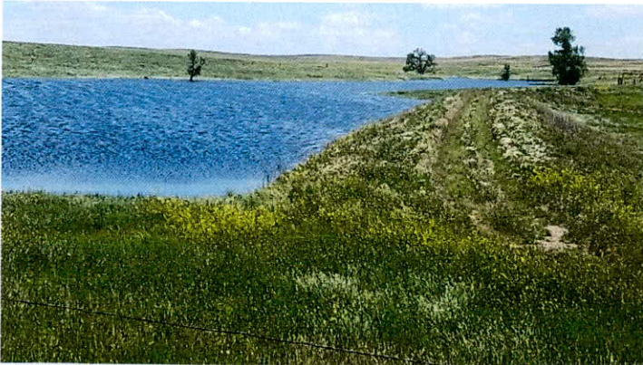
Dam embankment and pool (view to south)
