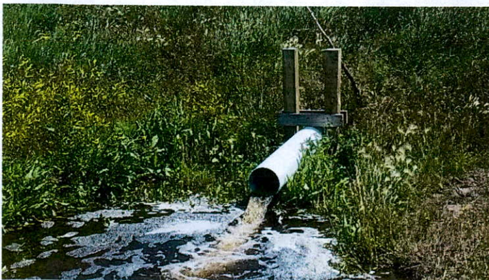
Principal Spillway at outlet
