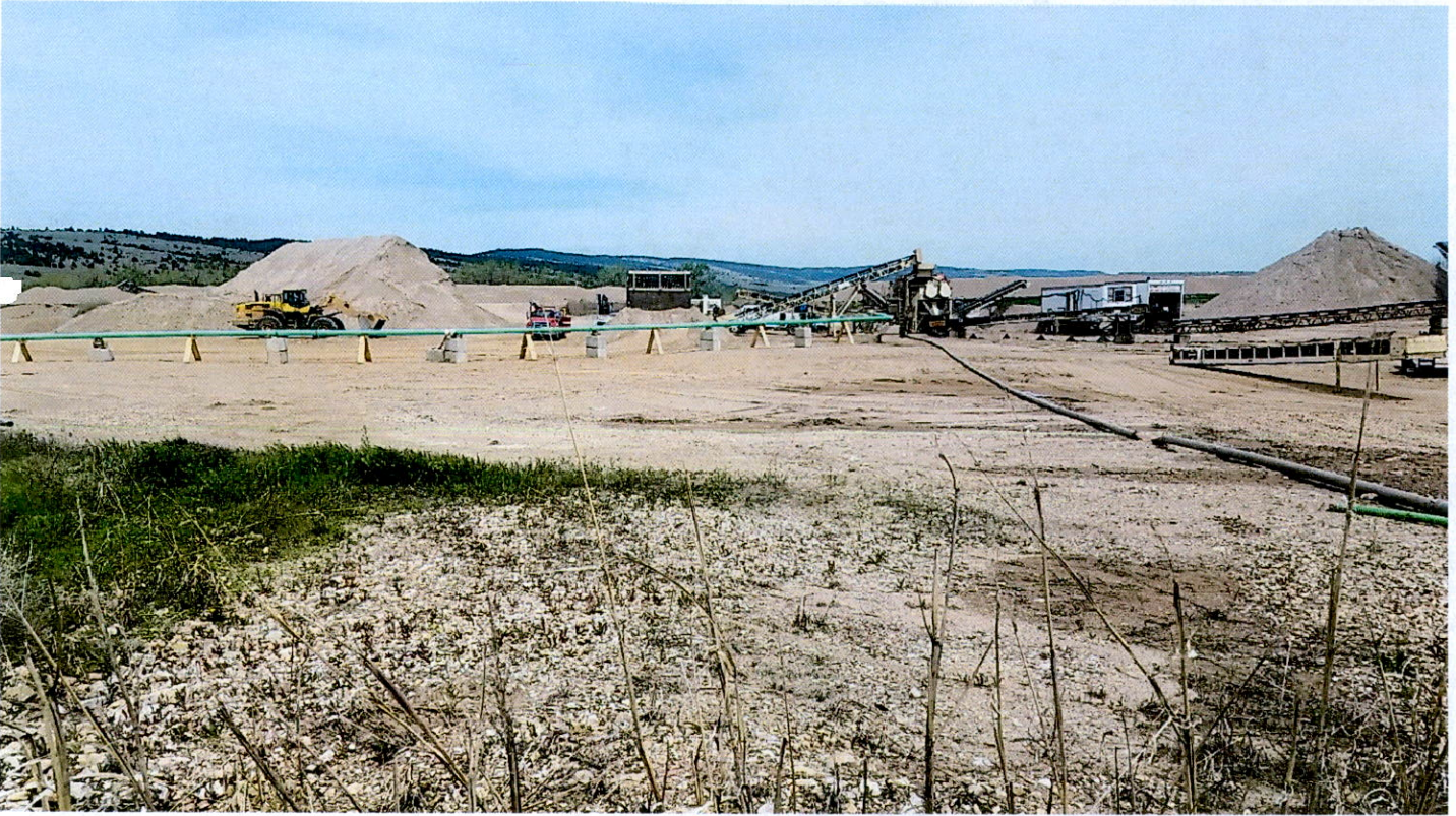
Gravel wash operation
