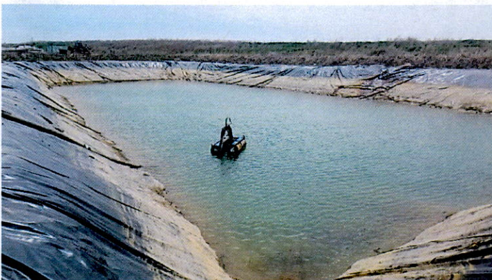
PVC lined storage pond for gravel wash operation
