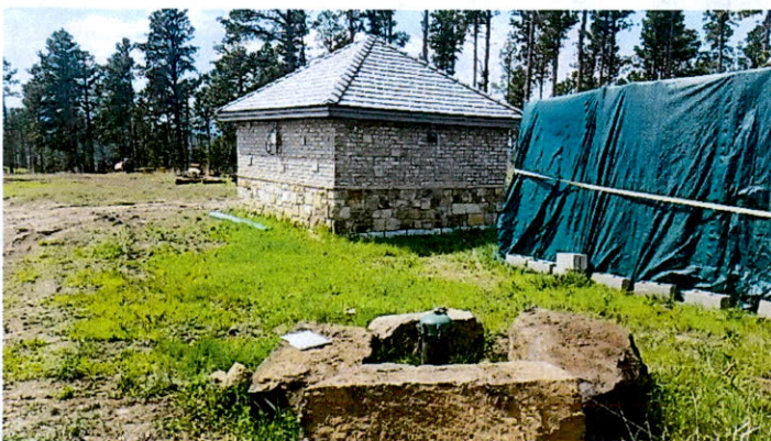
Well and pump house
