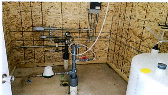
Pump house appurtenances
