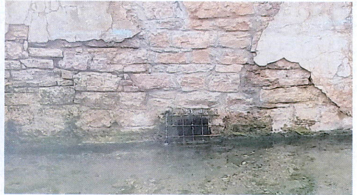
Discharge to city storm sewer through original 1890 wall.
