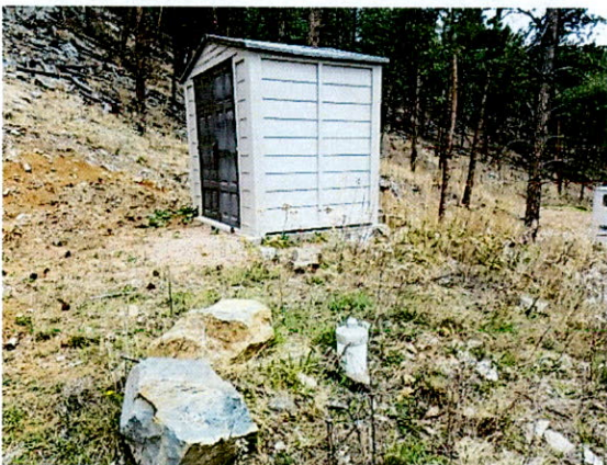
Well and pump house
