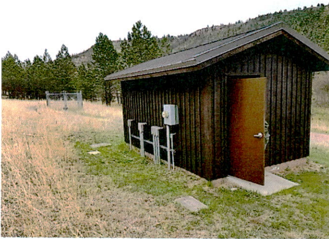
Pump house – 2001 well background (old well #2)
