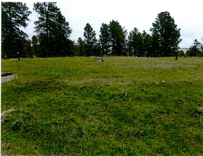
487,090 gallon underground concrete reservoir
