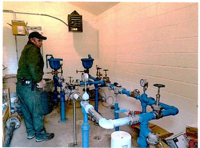
Pump house appurtenances
