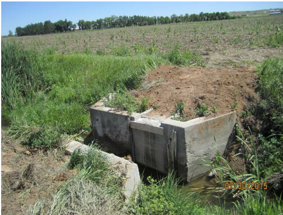
Figure 3-56. Turnout D Associated With Permit 2415-2. Headgate removed and concrete plug put in place for south turnout. Date 7/30/2015
