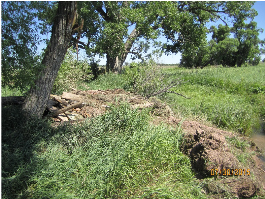
Figure 3-51. Turnout A Wooden Flume Structure Associated With Permit 2415-2, removed. Date 7/30/2015
