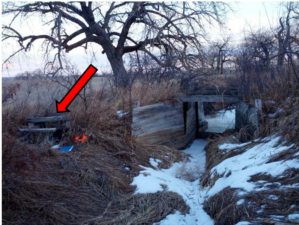
Figure 3-44. Turnout B (Red Arrow) and the Flume Associated with Permit 2415-2.
