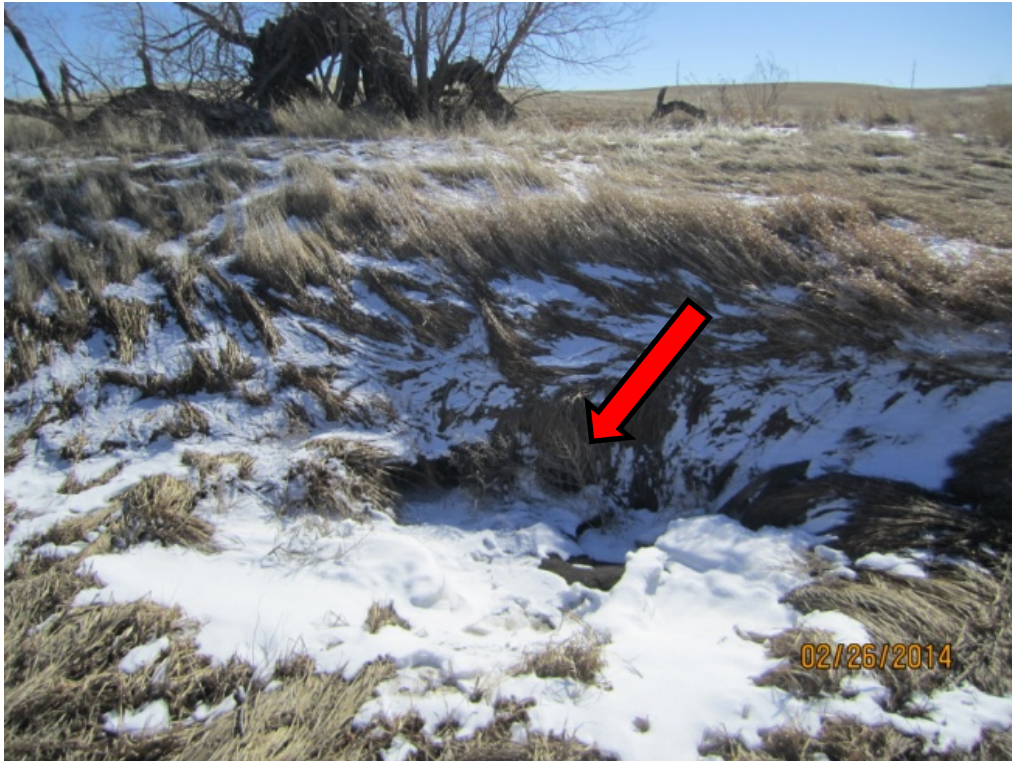
Figure 3-30. Outlet end of Turnout B pipe (Red Arrow). (Looking South, Towards South Side Ditch).
