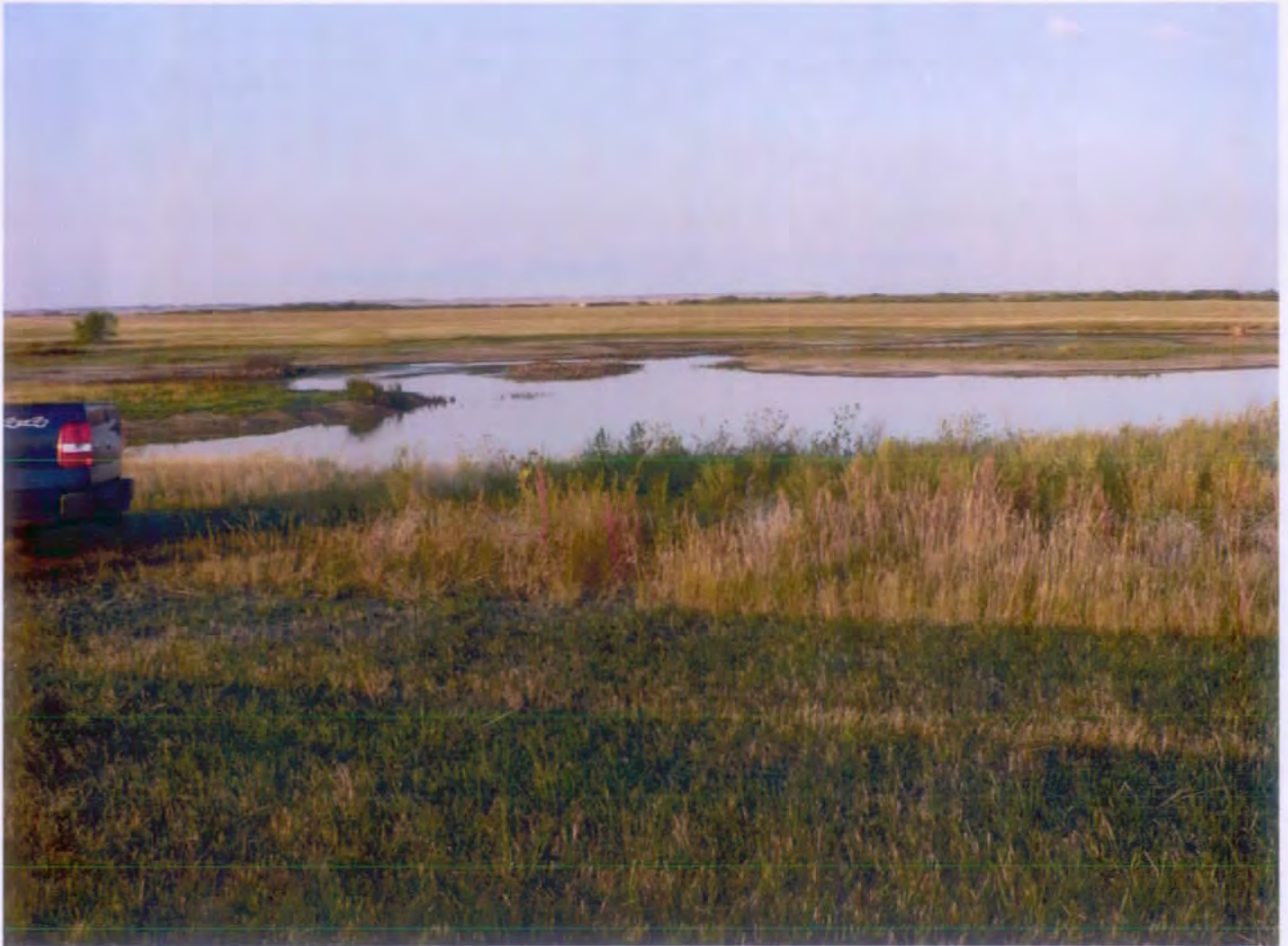
Picture taken along west edge of dam grade showing the relatively low level of the dam
