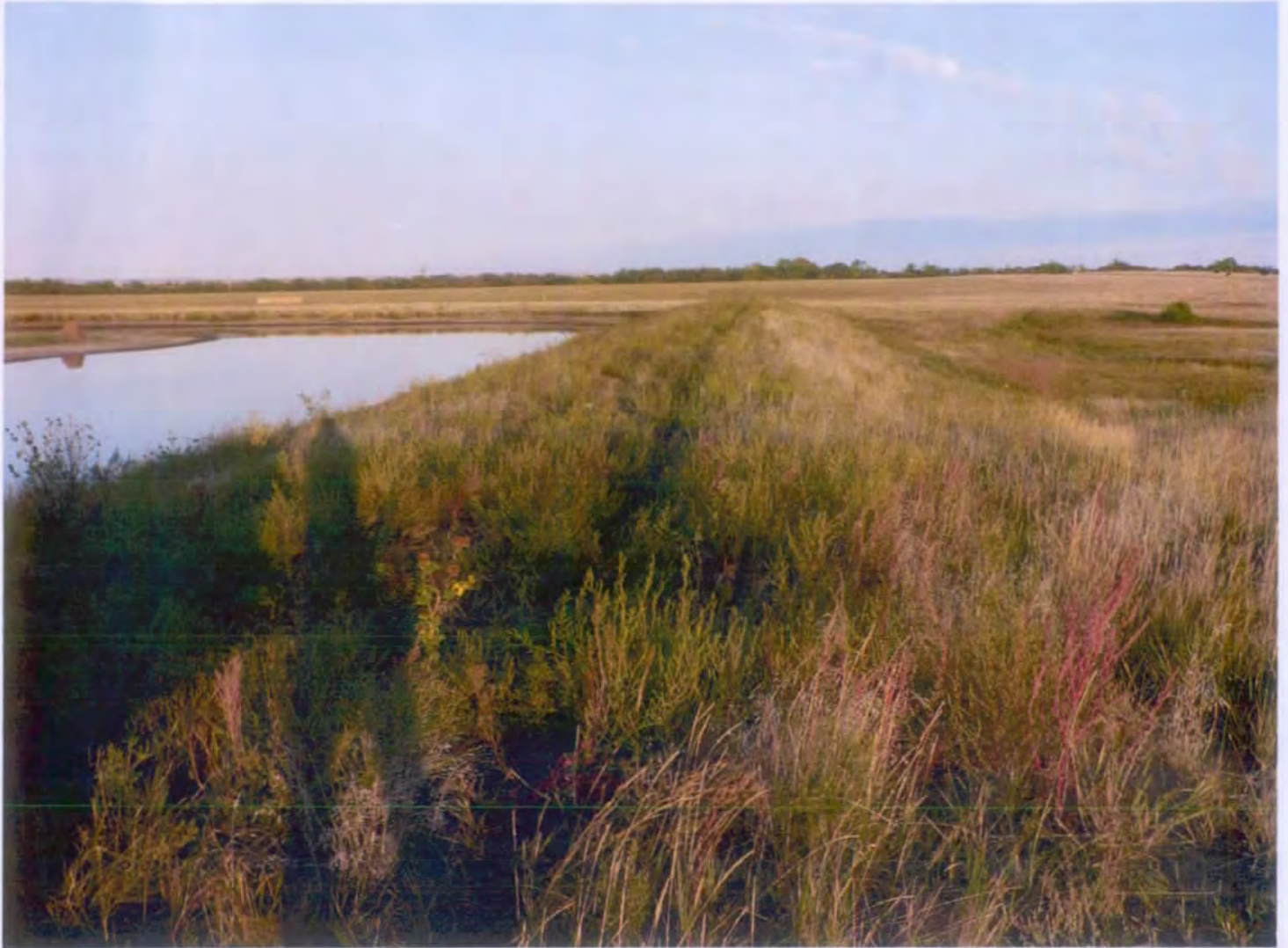
Picture of the dam grade looking in a westerly direction
