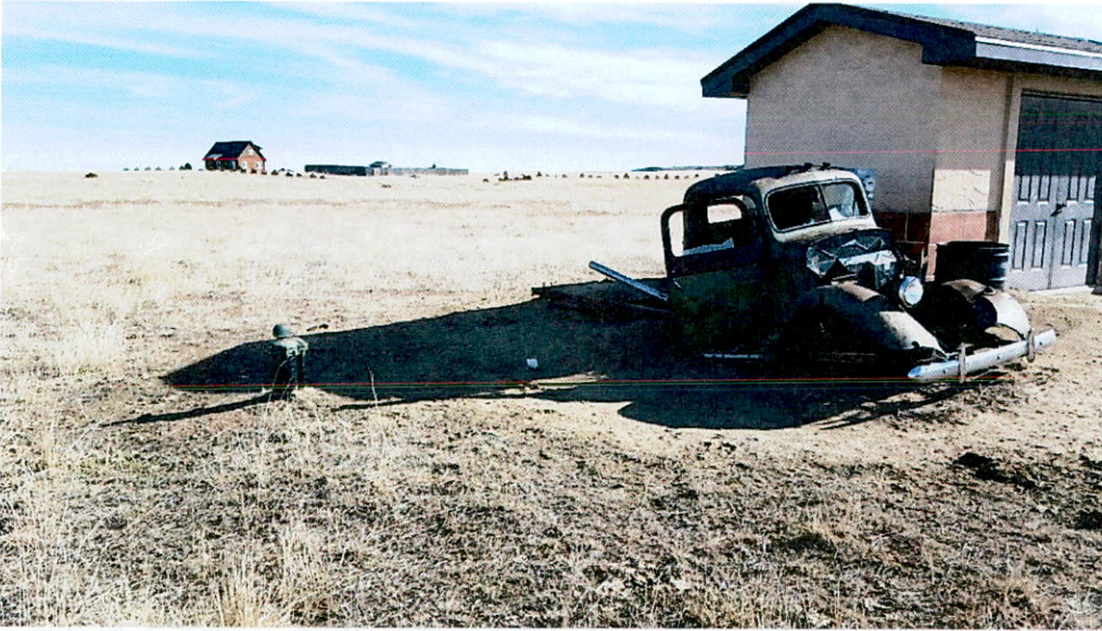
SD Lake LLC well and pump house
