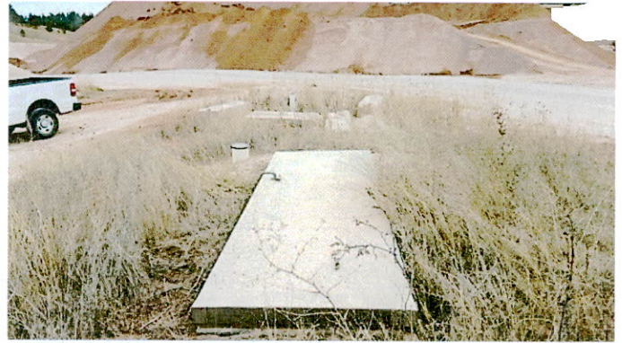
SBHWS booster pit with Streeter well in background
