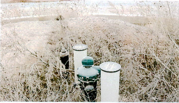
Streeter well after casing reconstructed to terminate above ground per SD well construction standards
