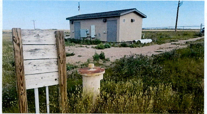
Well and pump house
