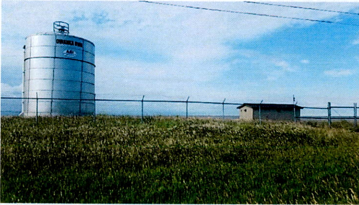
Storage and pump house
