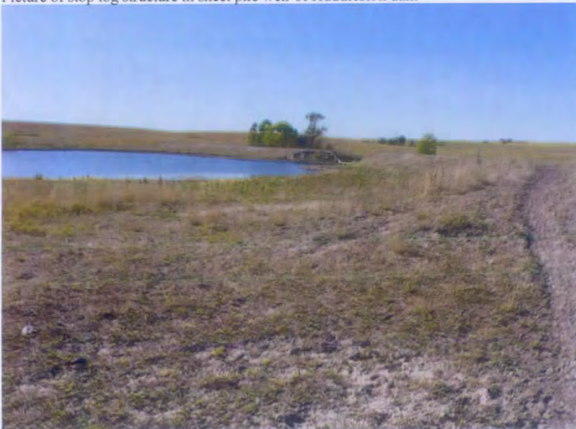
Picture looking in a westerly direction of the grade for Huddleston dam on Pass Creek
