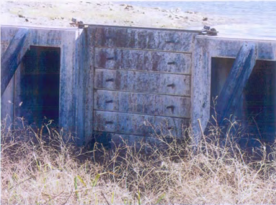
Picture of stop log structure in sheet pile weir of Huddleston dam
