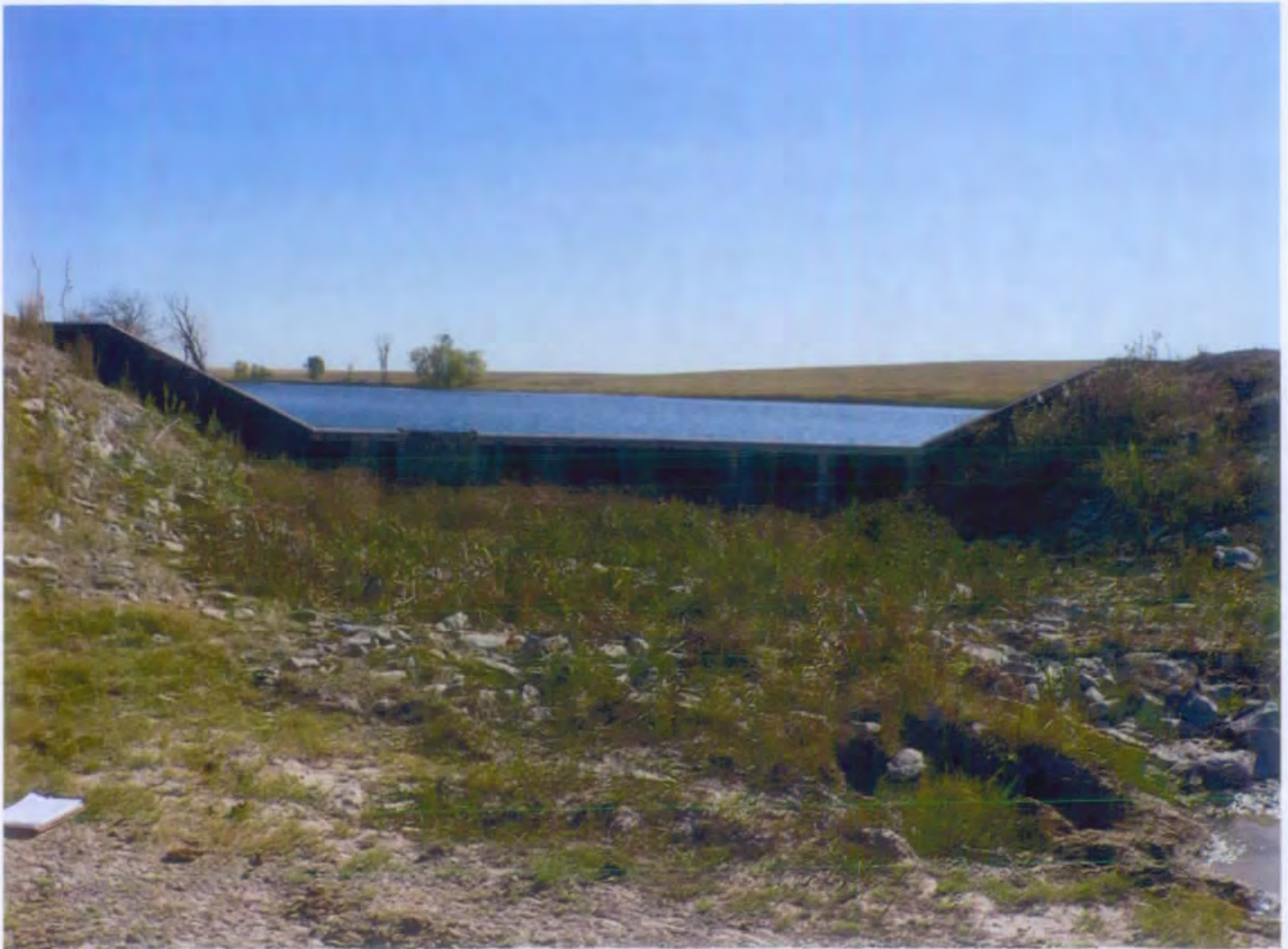
Sheet pile weir primary outlet of Huddleston dam – Permit No. 2611-2. Picture taken looking south.
