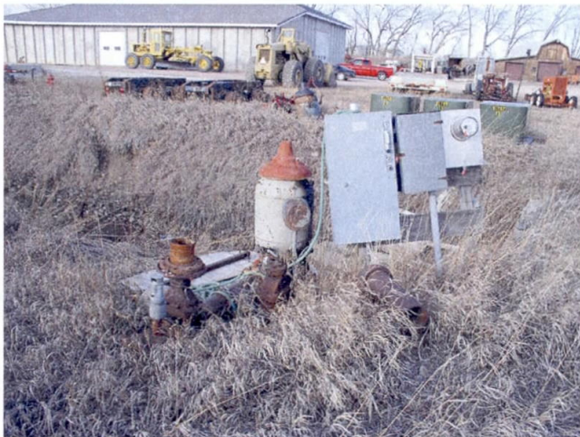
Northeast Pump Station
