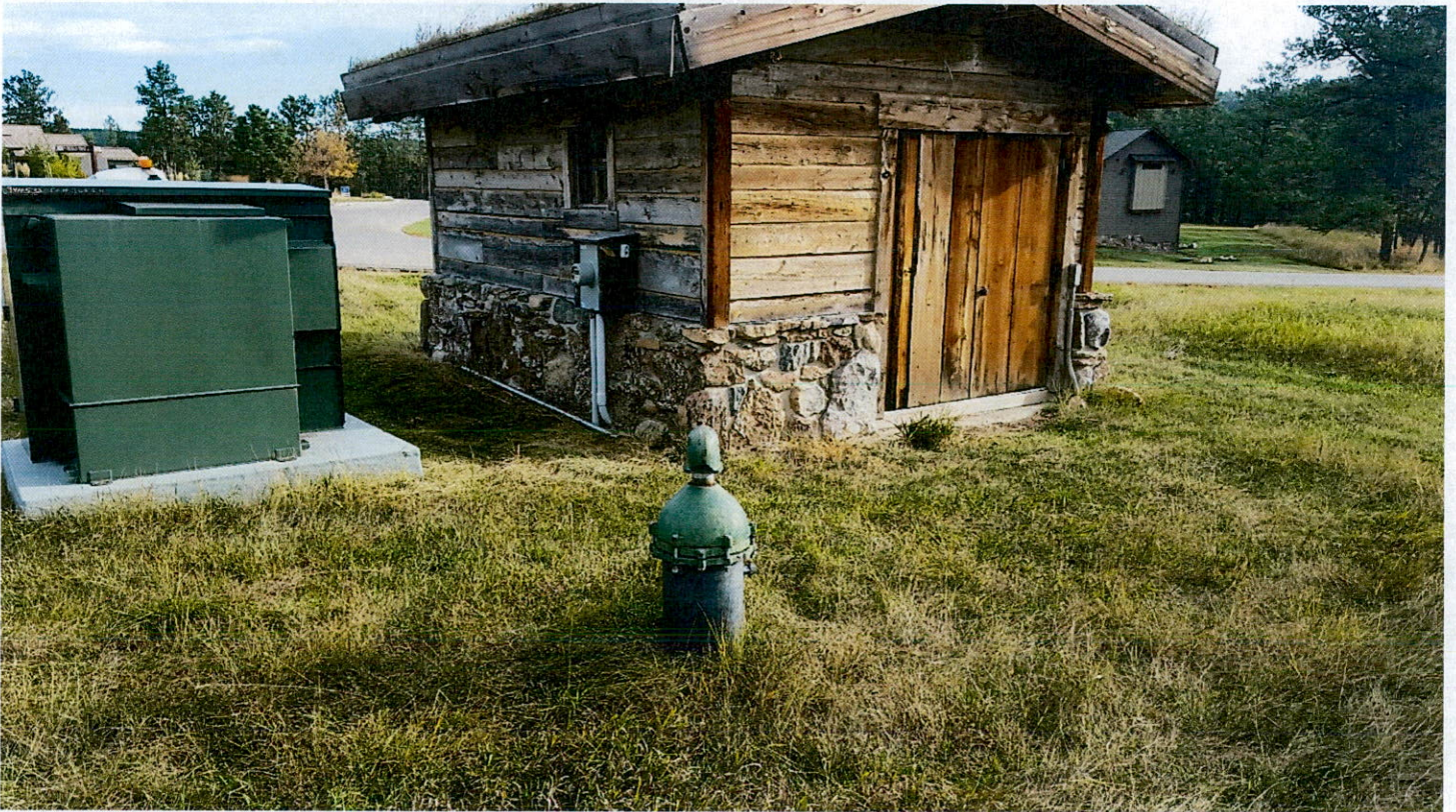
Canyon Springs Sanitary & Water District Well.
