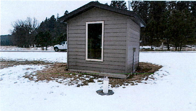
Well # 1 – Water Supply for Sheridan Lake Highlands
