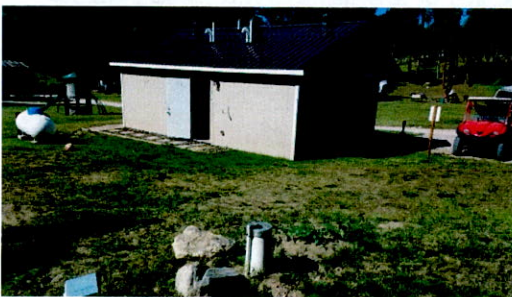
Well and pump/shower house
