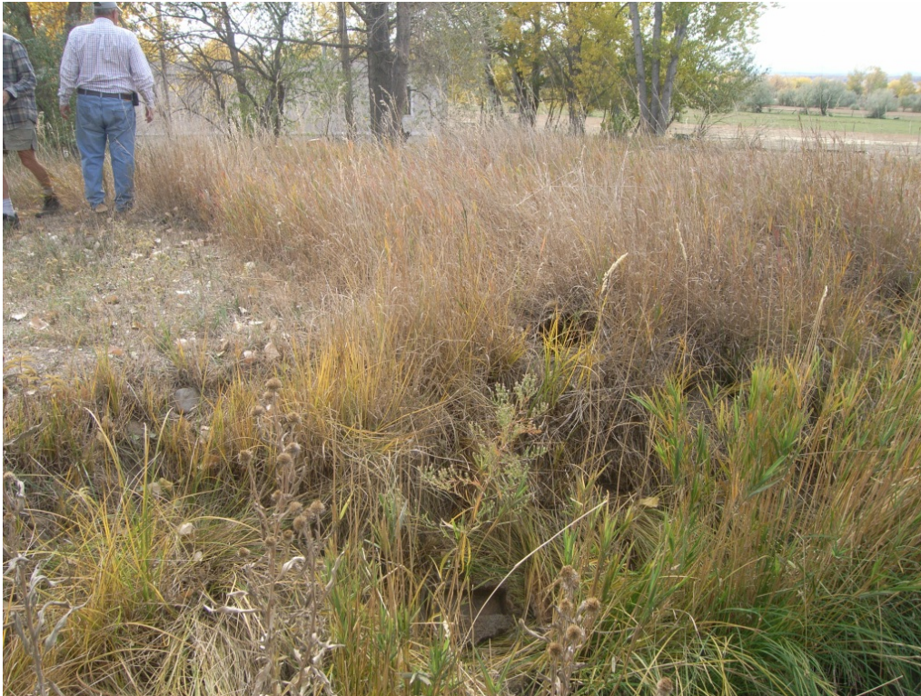
Figure 3-10. Photograph Taken From in the Murphy Ditch Running Right to Left (Bank in Foreground Is Likely Former Turnout Location for Permit 2201-2).
