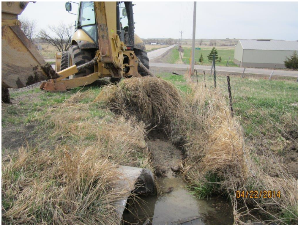
Figure 3-14. Removal of Turnout B for Permit 2399-2 Located on Murphy Ditch on Radar Road. Date 4/22/2014
