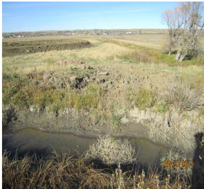
Figure 3-36. Turnout B Associated with Permit 2249-2. The old turnout structure has been removed. Date 10/29/2015.
