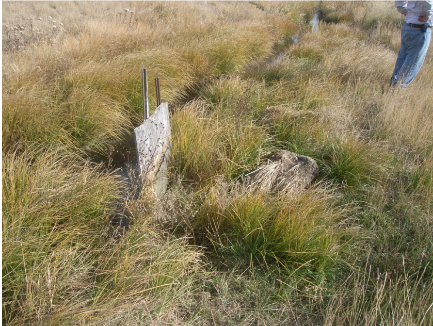
Figure 3-19. Plywood Headgate for Turnout B of Permit 2512-2.
