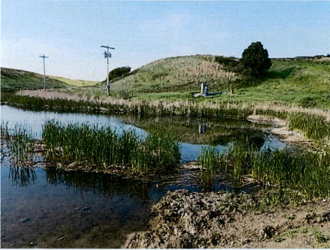
dam impoundment and pump from embankment
