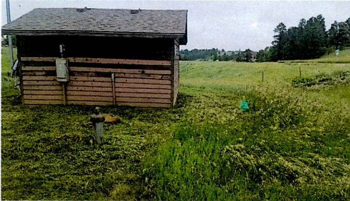
Dakota Aquifer well, the Minnelusa well is located 20' to the east and is hidden by tall grass.
