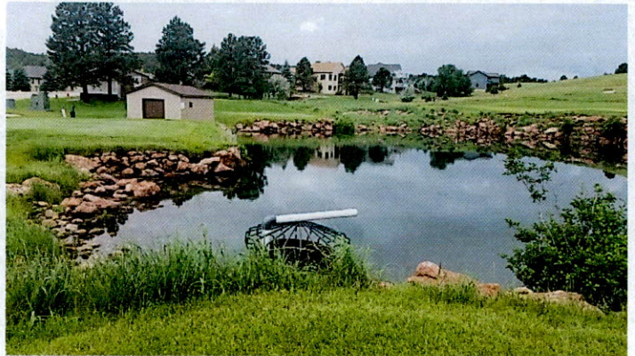
PVC supply from Dakota and Minnelusa wells discharging into storage pond. Metal trash rack and riser is overflow structure for pond. Pump house is situated at side of pond.
