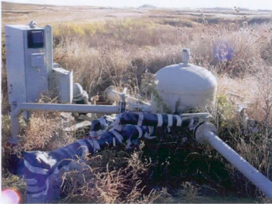
Little White River Diversion No. 1 (well well design – can see vertical motor in background) The primary focus of this picture is the manifold system by which the permit holder can direct water to the pond or for irrigation of the trees as they desire.
