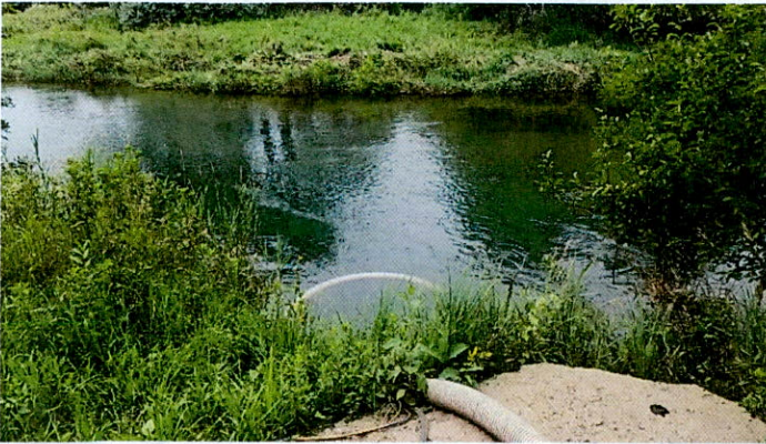
Rapid Creek diversion
