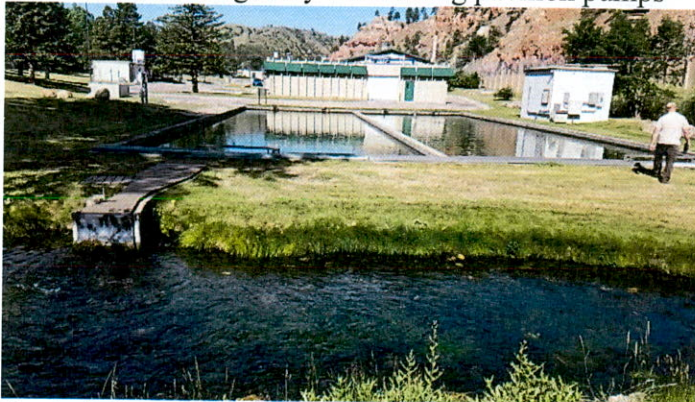
Parshall flume (left) and settling ponds
