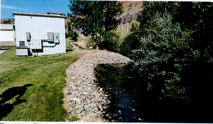
By-pass flow outlet to open channel
