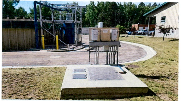
Hatchery building (upper left) and pump station
