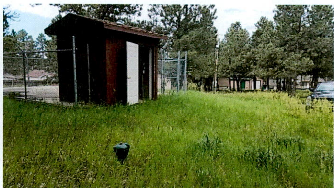
Well #2 and 40,000 gallon concrete storage and pump house
