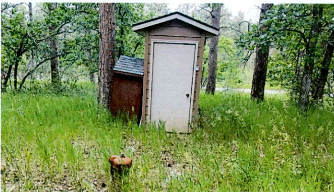
Well #1 and pump house
