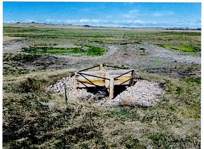
Principal Spillway inlet
