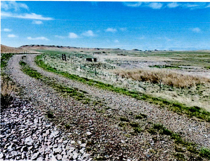
Dam crest on left, pool on right
