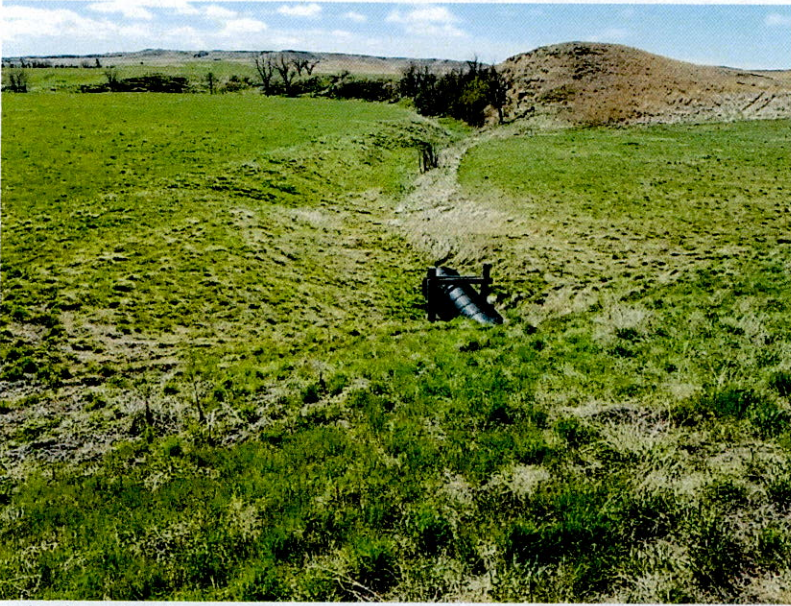
Principal Spillway outlet
