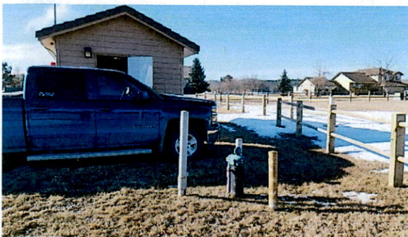
Well and pump house
