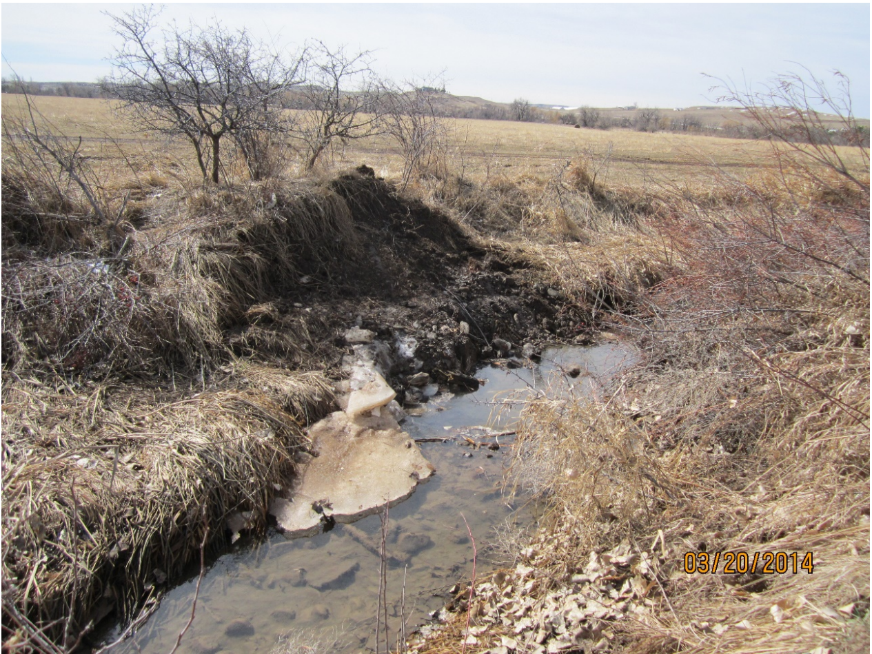
Figure 3-5. Removal of Turnout associated with Permit 2316-2. Date 3/20/2014
