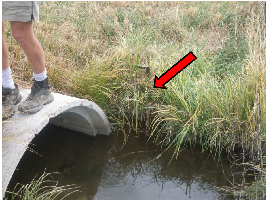
Figure 3-13. Turnout B for Permit 2399-2 (The 12-Inch Steel Canal Gate was Located on the Far Bank Adjacent to the Concrete Culvert, and Murphy Ditch Runs Right to Left).
