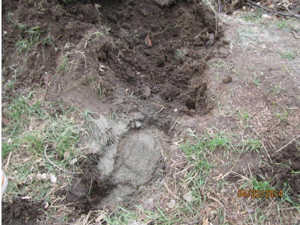
Figure 3-8. Removal of Turnout A Associated With Permit 2469-2. Date 4/22/2014
