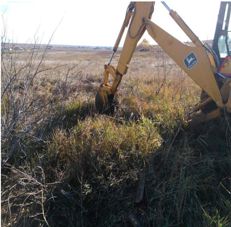
Figure 3-40. Turnout D Associated With Permit 2249-2. Photo of the division box being removed and backfilled by the City. Date 10/30/2015.
