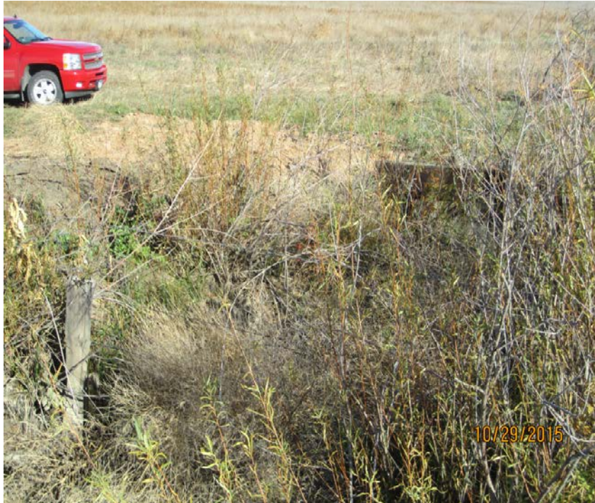
Figure 3-37. Turnout C Associated With Permit 2249-2. Removed turnout structure. Date 10/29/2015.
