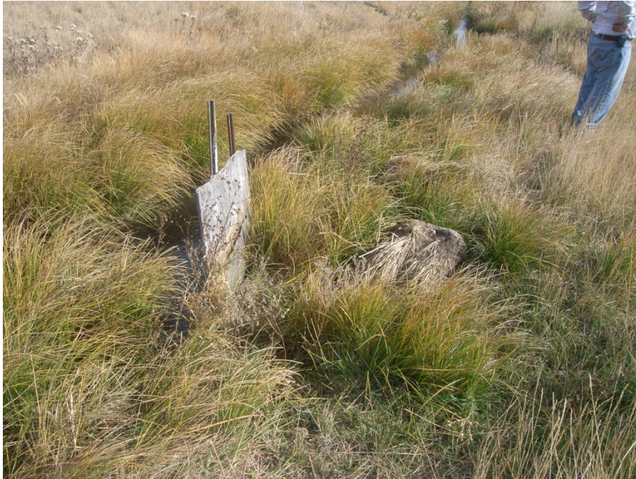
Figure 3-19. Plywood Headgate for Turnout B of Permit 2512-2.
