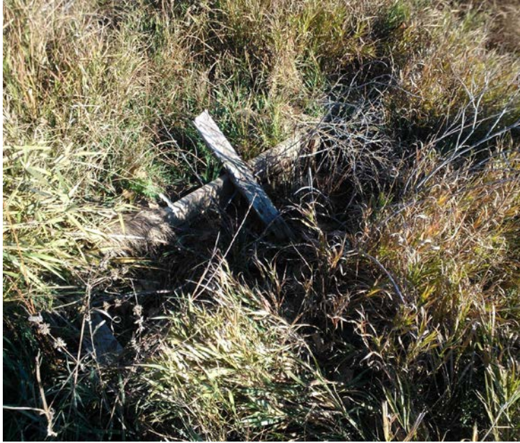
Figure 3-34. Turnout D Division Box Associated With Permit 2249-2. Date 10/30/2015.
