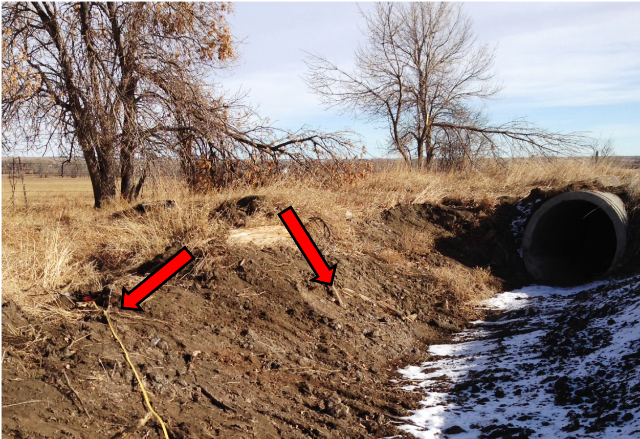
Figure 3-1. The Turnout Ditch (Left Arrow) and Former Location of Flume (Right Arrow) Associated With Permit 2655-2. Cyclone Ditch Runs From Foreground to Background Through Large Concrete Pipe.
