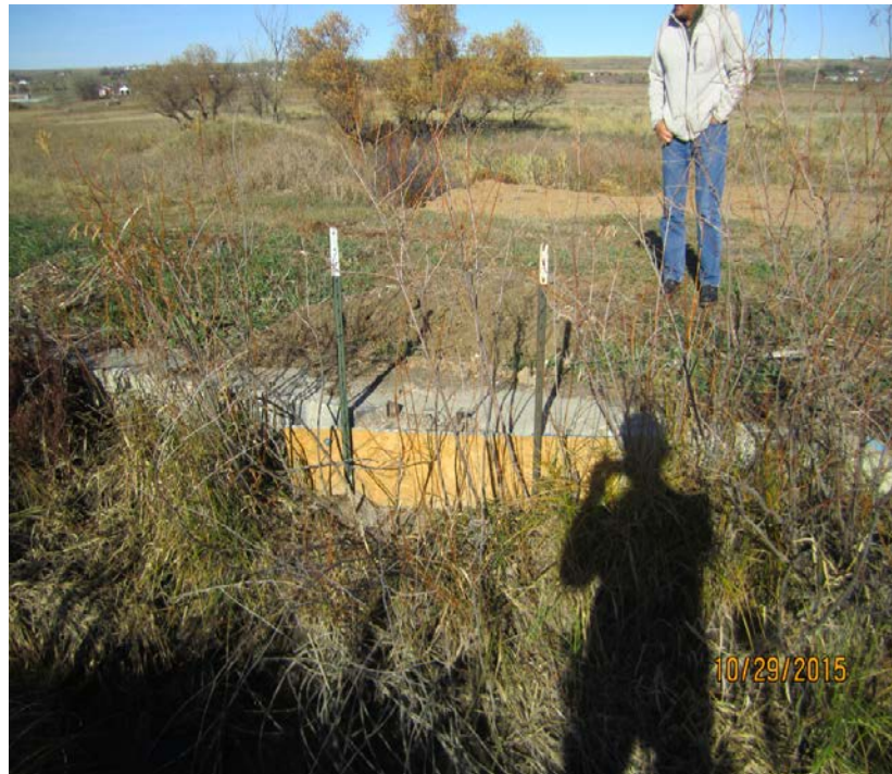
Figure 3-35. Turnout A Associated with Permit 2249-2. Headgate removed, turnout pipe filled with concrete, and outlet filled in. Date 10/29/2015
