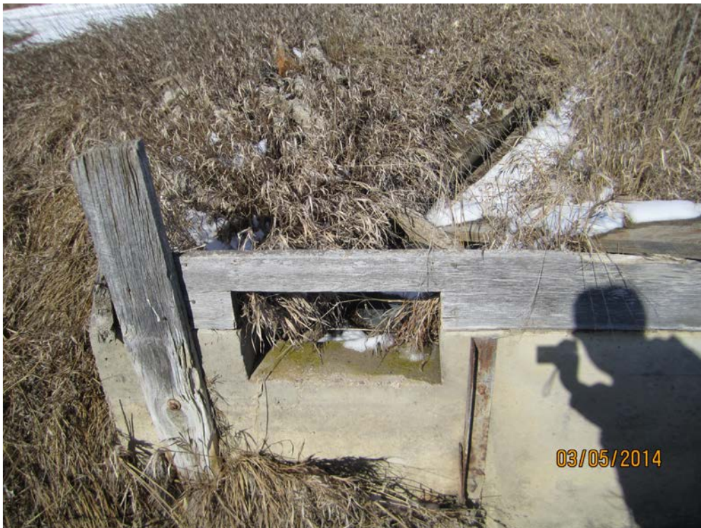
Figure 3-48. North Flume/Check Structure Wall and Outlet for Turnout D Associated With Permit 2415-2.
