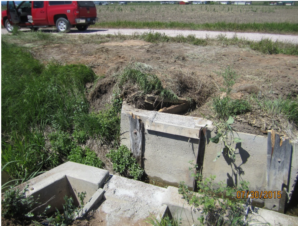
Figure 3-57. Turnout D Associated With Permit 2415-2. Headgate removed and concrete plug put in place for north turnout. Date 7/30/2015.
