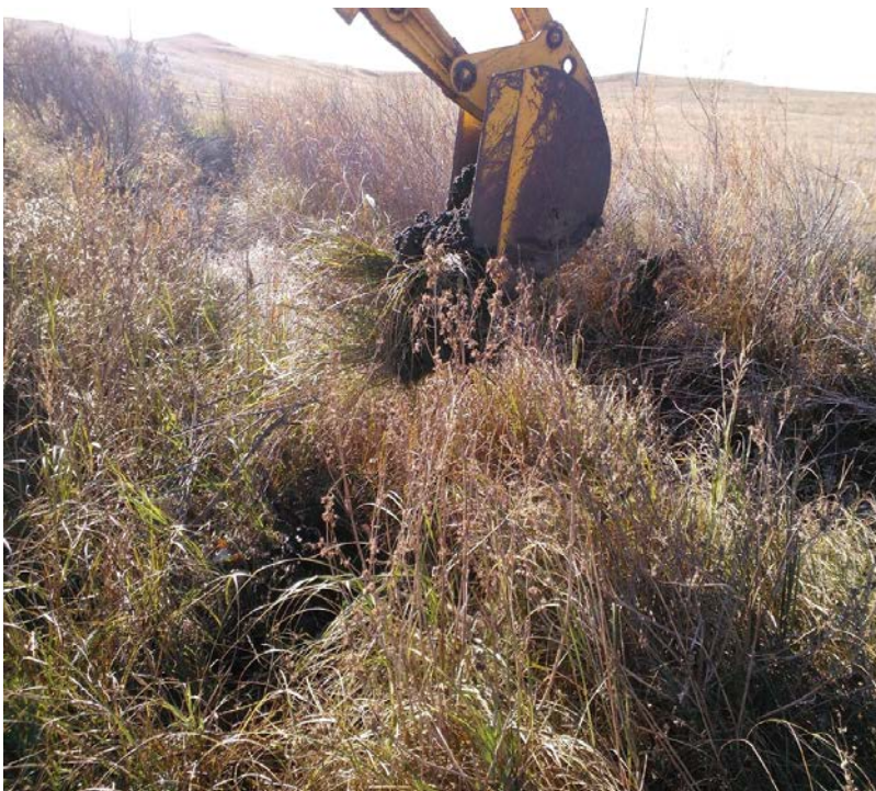
Figure 3-39. Turnout D Associated With Permit 2249-2. Turnout being backfilled. Date 10/30/2015.
