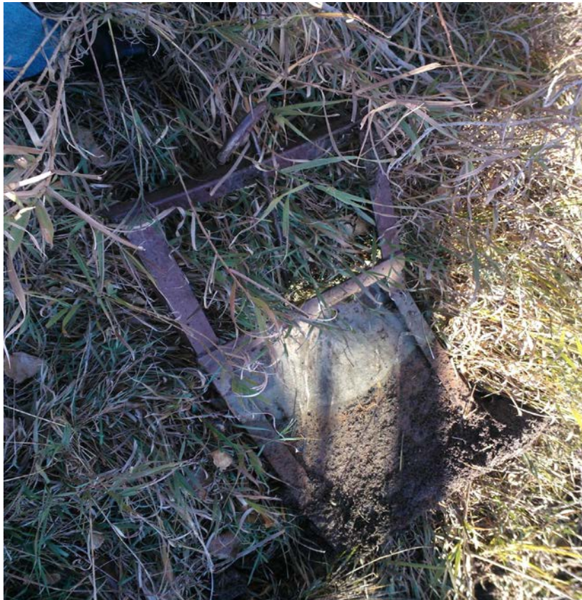
Figure 3-38. Turnout D Associated With Permit 2249-2, removed by the City. Date 10/30/2015
