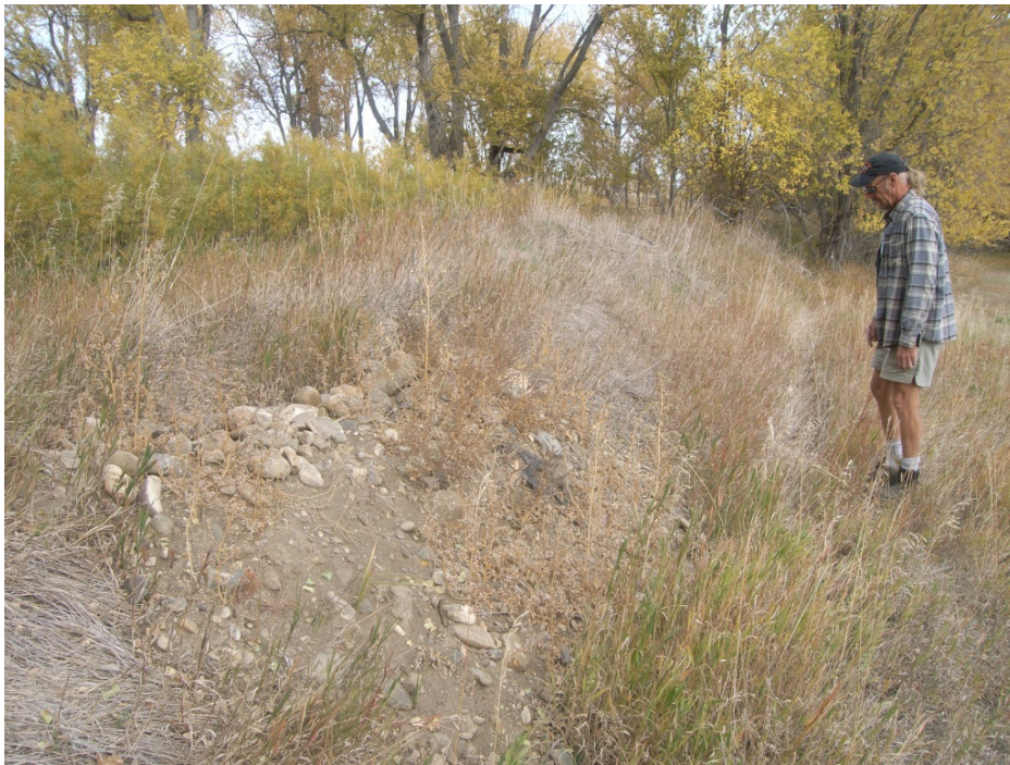
Figure 3-12. Backfill Material at the Former Location of Turnout A for Permit 2399-2. This area has since had material added to the bank.
