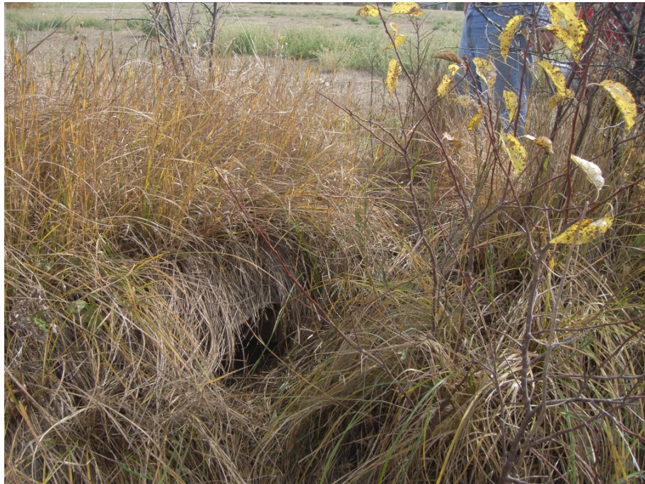
Figure 3-3. Opening to 12-Inch-Diameter Corrugated Metal Pipe Turnout for Permit 2316-2.
