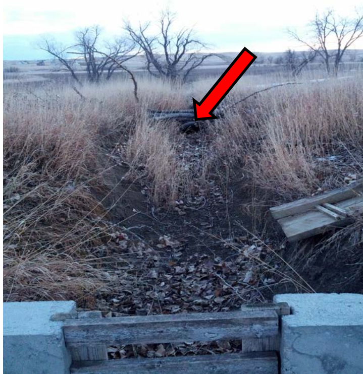
Figure 3-46. Turnout C and the 24-Inch-Diameter Concrete Pipe (Red Arrow) Associated With Permit 2415-2.
