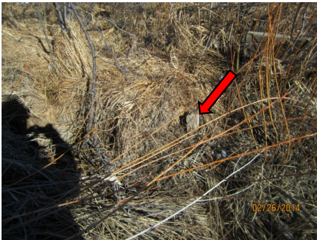
Figure 3-32. Wooden Structure (Red Arrow) for Turnout C Associated With Permit 2249-2. This structure is immediately upstream of the culvert crossing in Figure 3-31, on the north bank.
