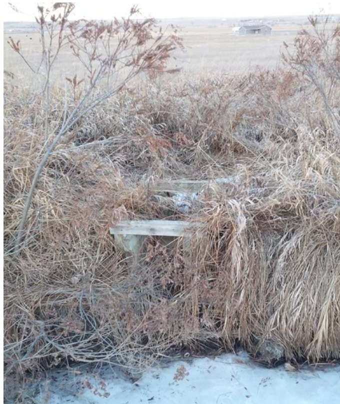
Figure 3-42. Turnout A for Permit 2415-2. The turnout is composed of timber.
