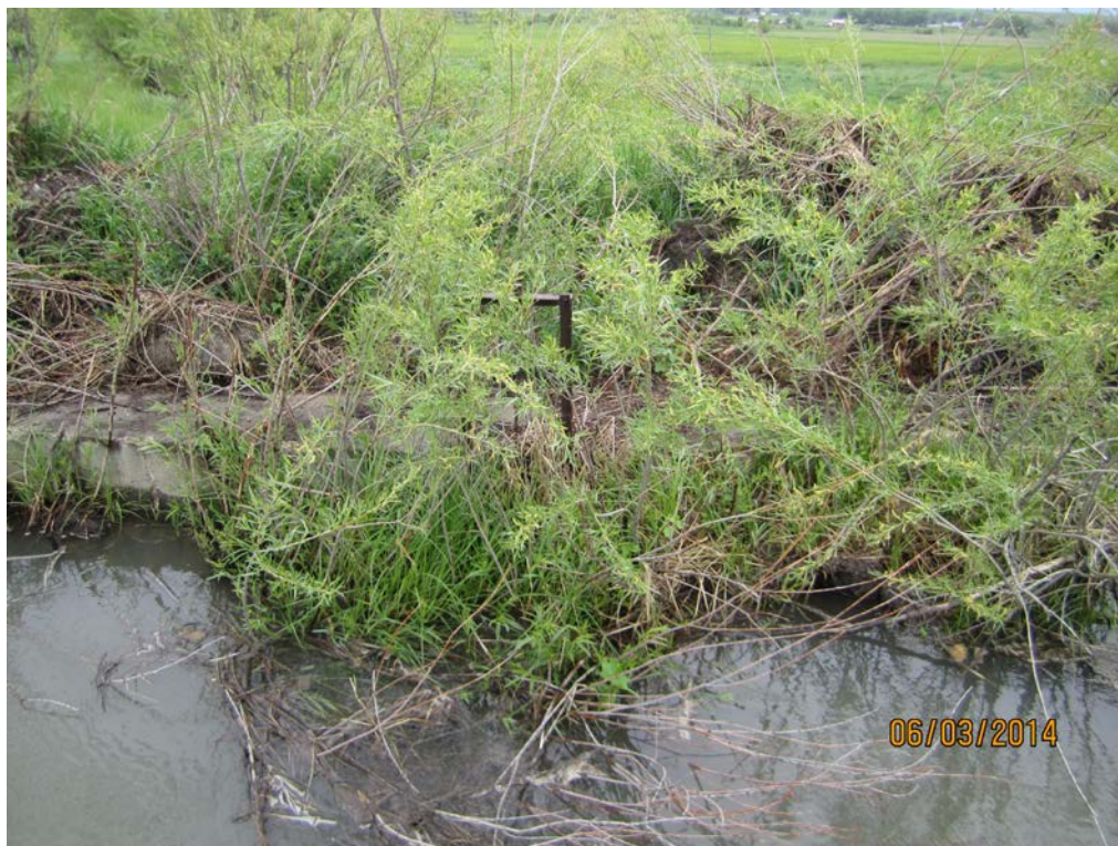
Figure 3-28. Turnout A structure Associated with Permit 2249-2.
