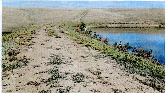
Crest of dam and pool
