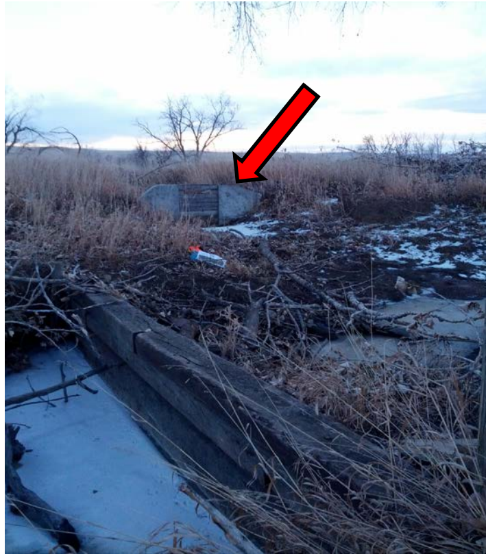
Figure 3-45. Turnout C (Red Arrow) and the Wooden Weir Associated With Permit 2415-2.
