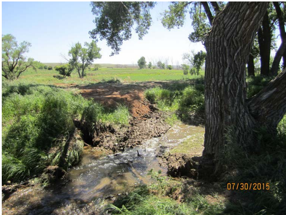
Figure 3-54. Turnout C Associated With Permit 2415-2 Timber Gate Turnout Structure, Concrete Abutments, and Timber Weir Check Structure Removed. Date 7/30/2015.
