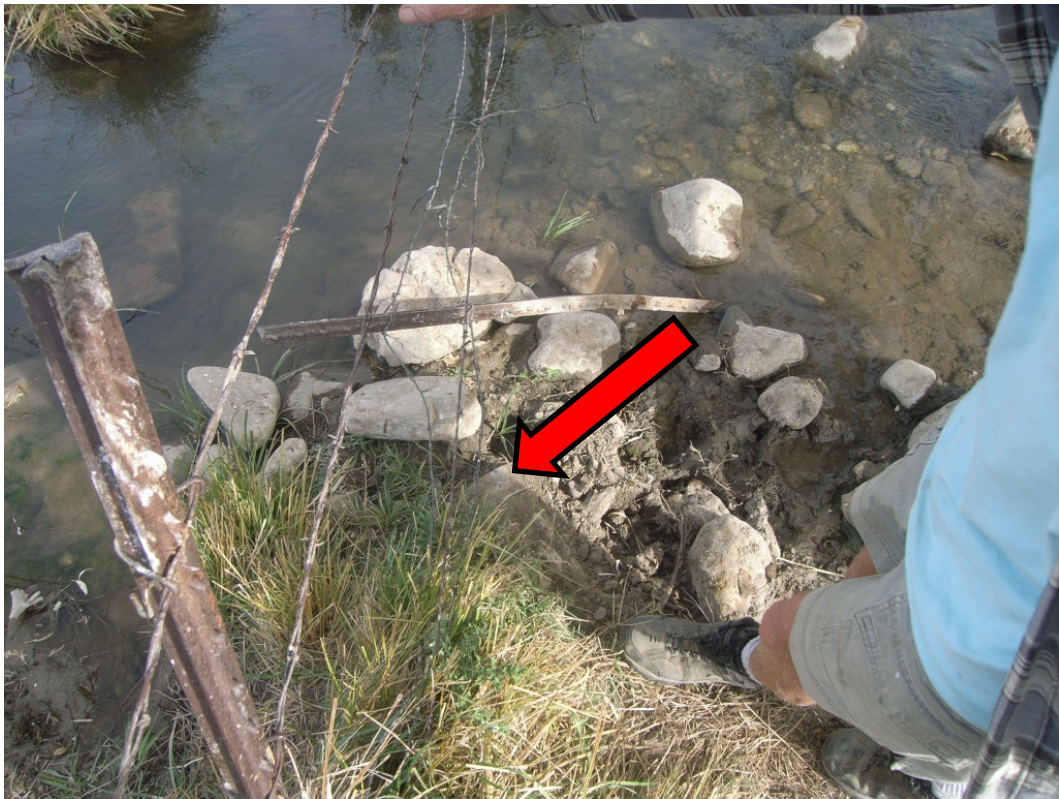
Figure 3-18. Pipe Used for Turnout A of Permit 2512-2 (Red Arrow).
