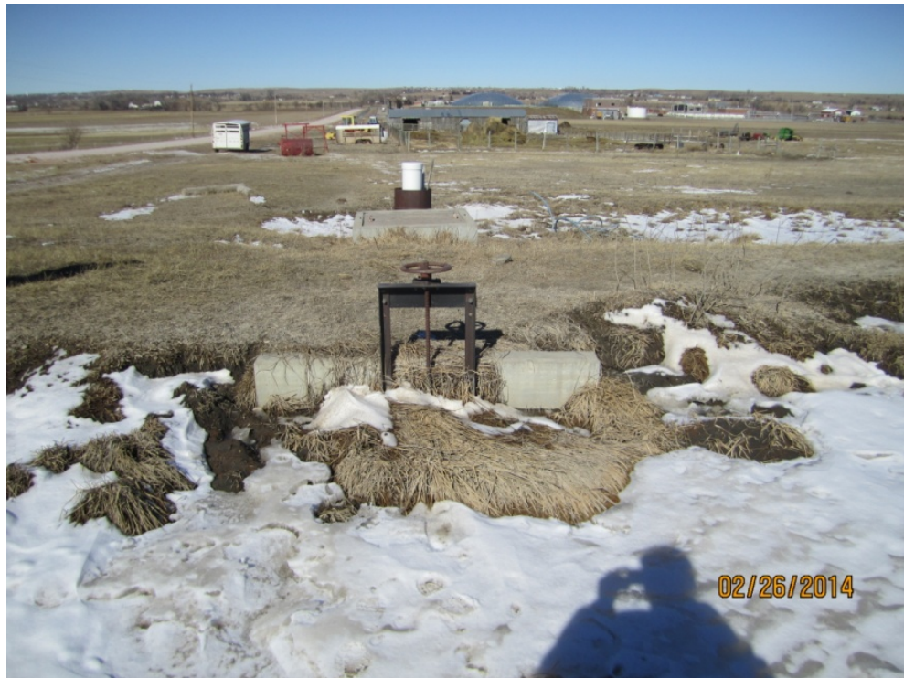
Figure 3-24. Inlet Structure, Weir Box, and Air Vent Associated With Turnout 2513-2.
