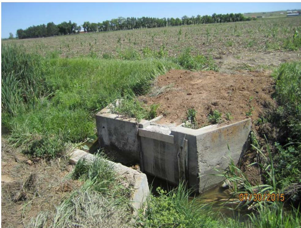
Figure 3-56. Turnout D Associated With Permit 2415-2. Headgate removed and concrete plug put in place for south turnout. Date 7/30/2015
