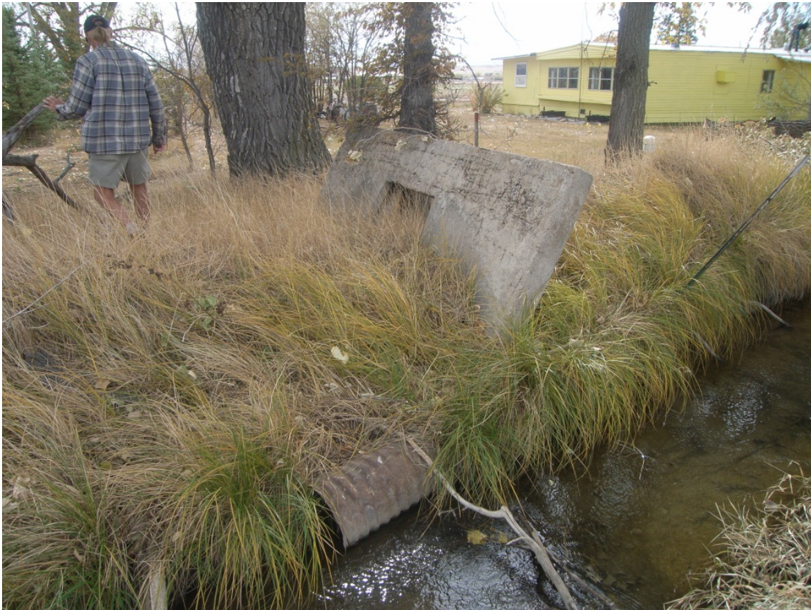
Figure 3-17. Former Location of the Turnout for Permits 2142-2 and 2199-2 (The Concrete Check Structure and a Disconnected Corrugated Metal Pipe Segment Sit on the Far Bank, and Murphy Ditch Flows Right to Left).
