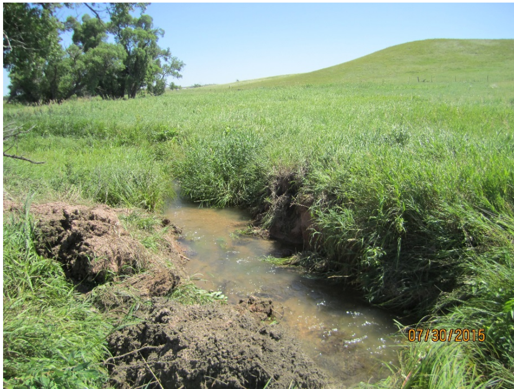
Figure 3-50. Removal of Turnout A associated with Permit 2415-2. Date 7/30/2015
