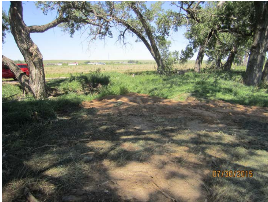
Figure 3-55. Turnout C Associated With Permit 2415-2. Turnout ditch filled in. Date 7/30/2015.
