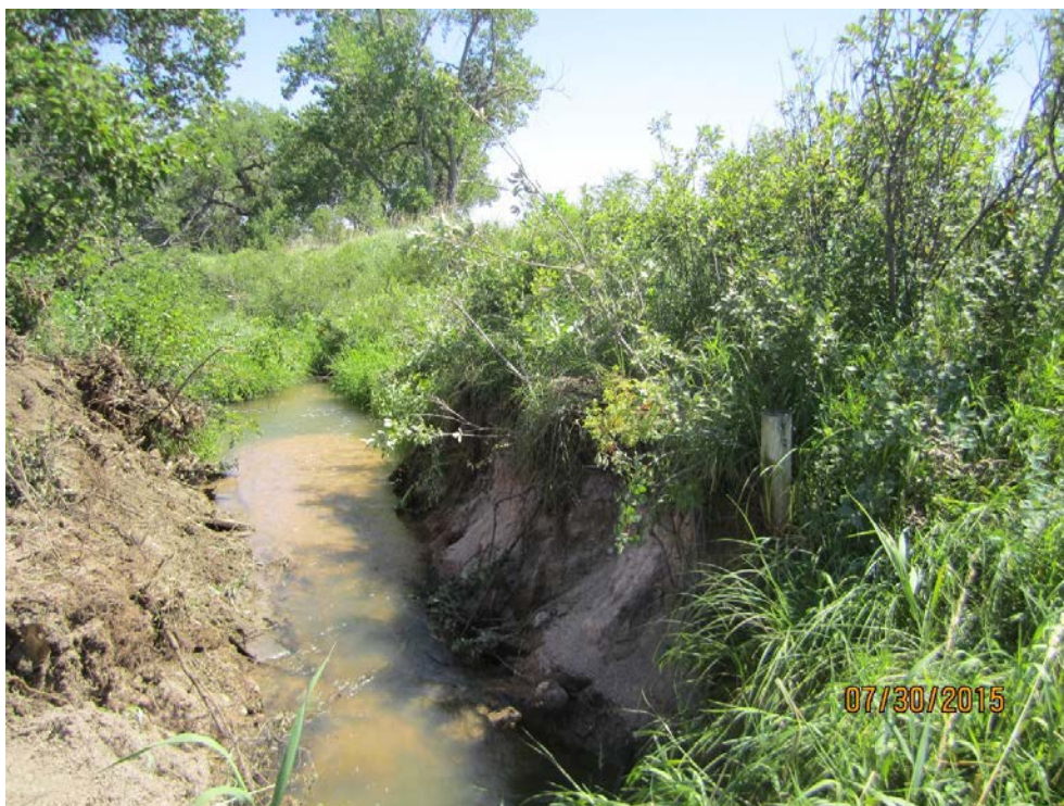
Figure 3-53. Turnout B Associated With Permit 2415-2. Wooden Flume Structure Removed. Date 7/30/2015.
