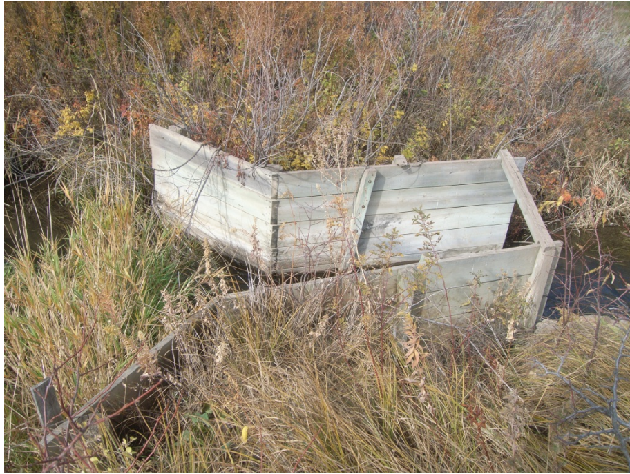
Figure 3-2. Wooden Flume Used as a Check for Permit 2316-2.
