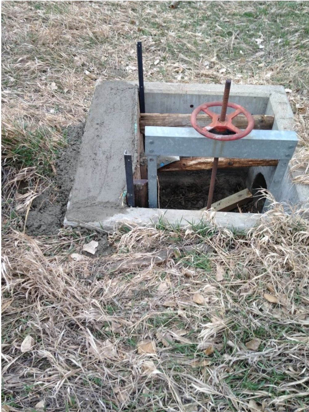
Figure 3-22. Removal of Turnout C for Permit 2512-2 Located on Murphy Ditch on the East Side of Airport Road Going South to the Airport. Date 4/22/2014.
