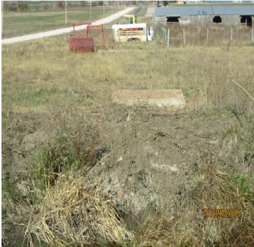
Figure 3-27. Removal of Turnout for Permit 2513-2. Headgate removed, measurement box filled with dirt and pipeline air vent removed. Date: 10/29/2015
