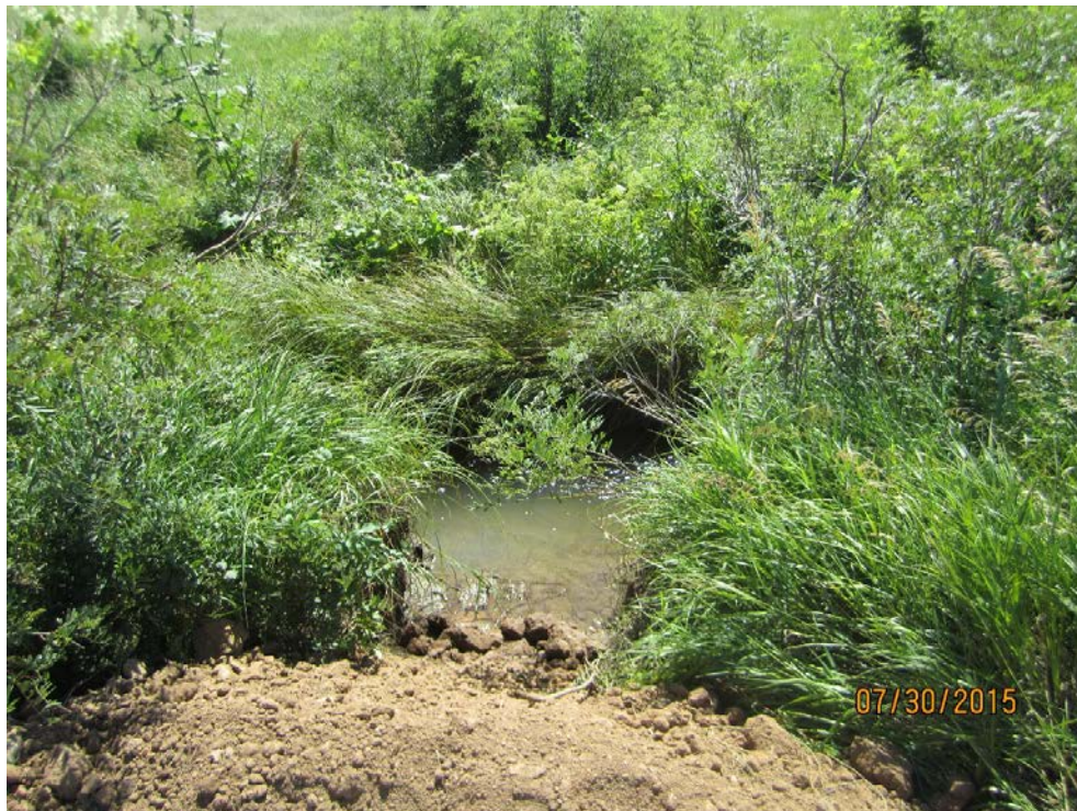
Figure 3-52. Turnout B Associated With Permit 2415-2. Timber Turnout Removed. Date 7/30/2015.
