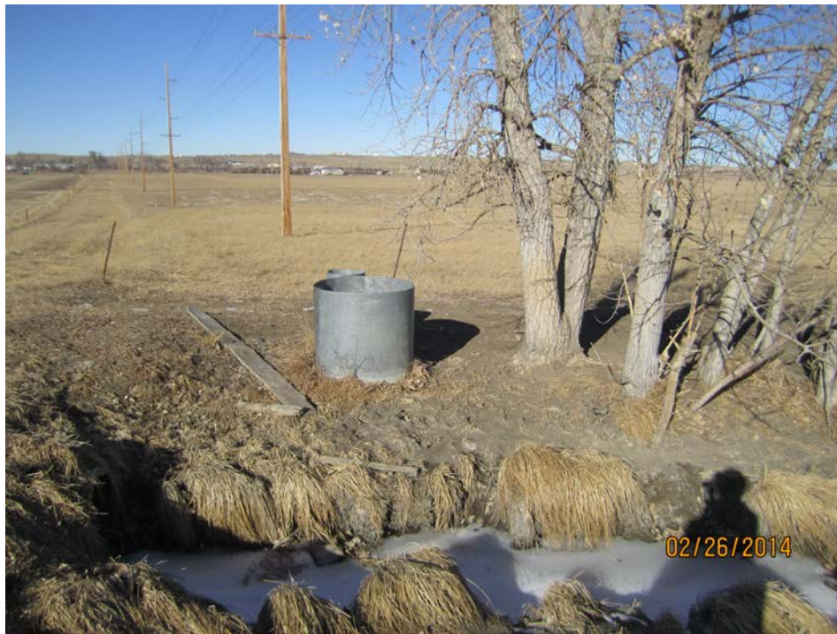
Figure 3-41. Turnout for Permit 2218-2. This turnout has been disabled and will not be disturbed.
