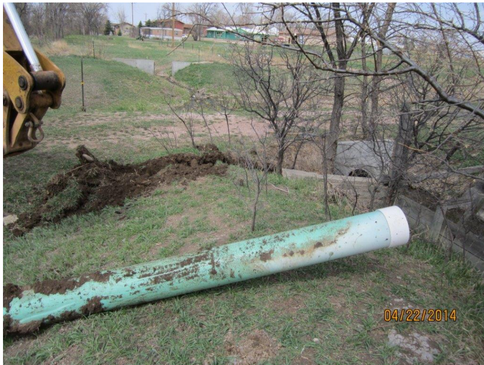
Figure 3-9. Removal of Turnout B Associated With Permit 2469-2. Date 4/22/2014.
