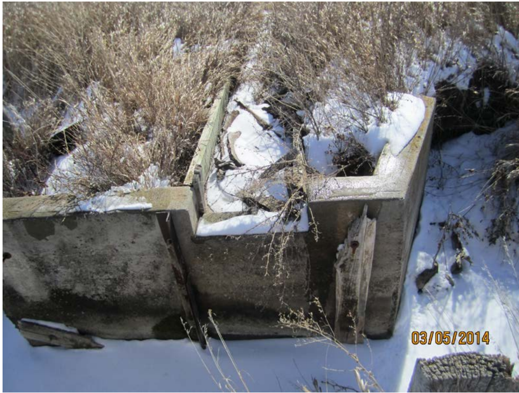
Figure 3-49. South Flume/Check Structure Wall and Outlet for Turnout D Associated With Permit 2415-2.
