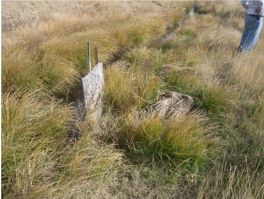
Figure 3-19. Plywood Headgate for Turnout B of Permit 2512-2.
