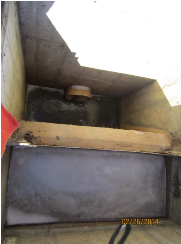
Figure 3-26. Inside the Weir Box for Turnout 2513-2. Note center wall weir and PVC pipe exiting the box.
