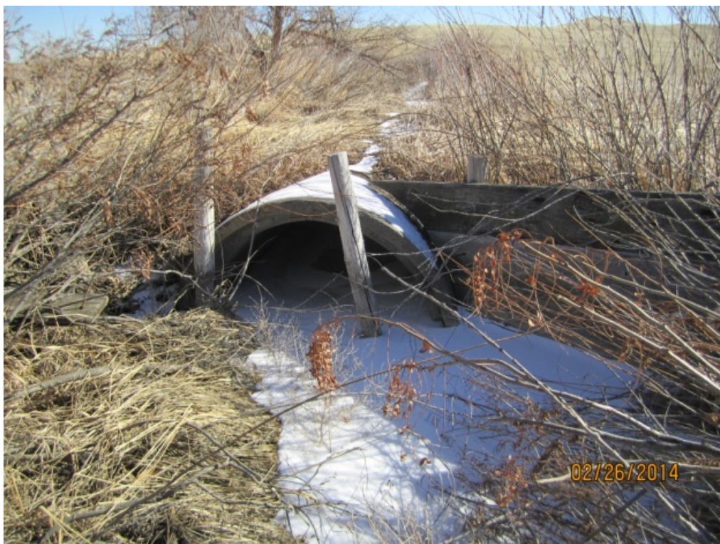
Figure 3-29. Culvert Crossing Used as a Check for Turnout B Associated with Permit 2249-2.
