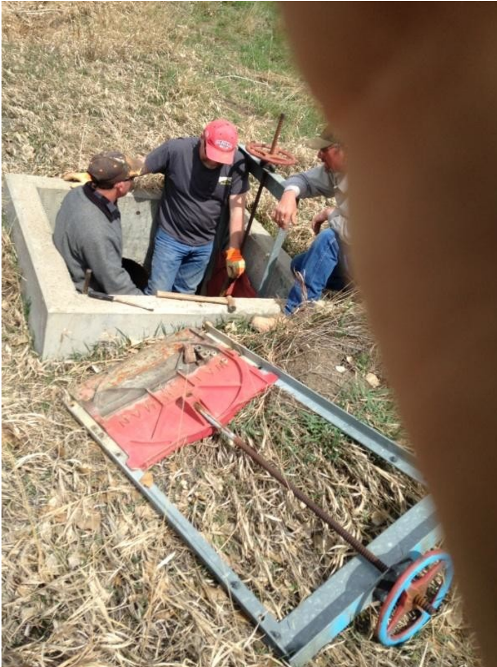
Figure 3-21. Removal of Turnout C for Permit 2512-2 Located on Murphy Ditch on the East Side of Airport Road. Date 4/22/2014
