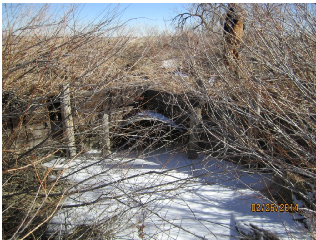
Figure 3-31. Second Culvert Crossing, Used as Check for Turnout C Associated With Permit 2249-2.
