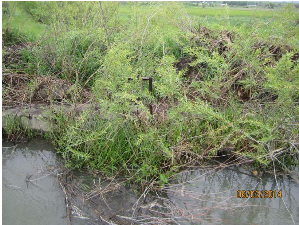
Figure 3-28. Turnout A structure Associated with Permit 2249-2.
