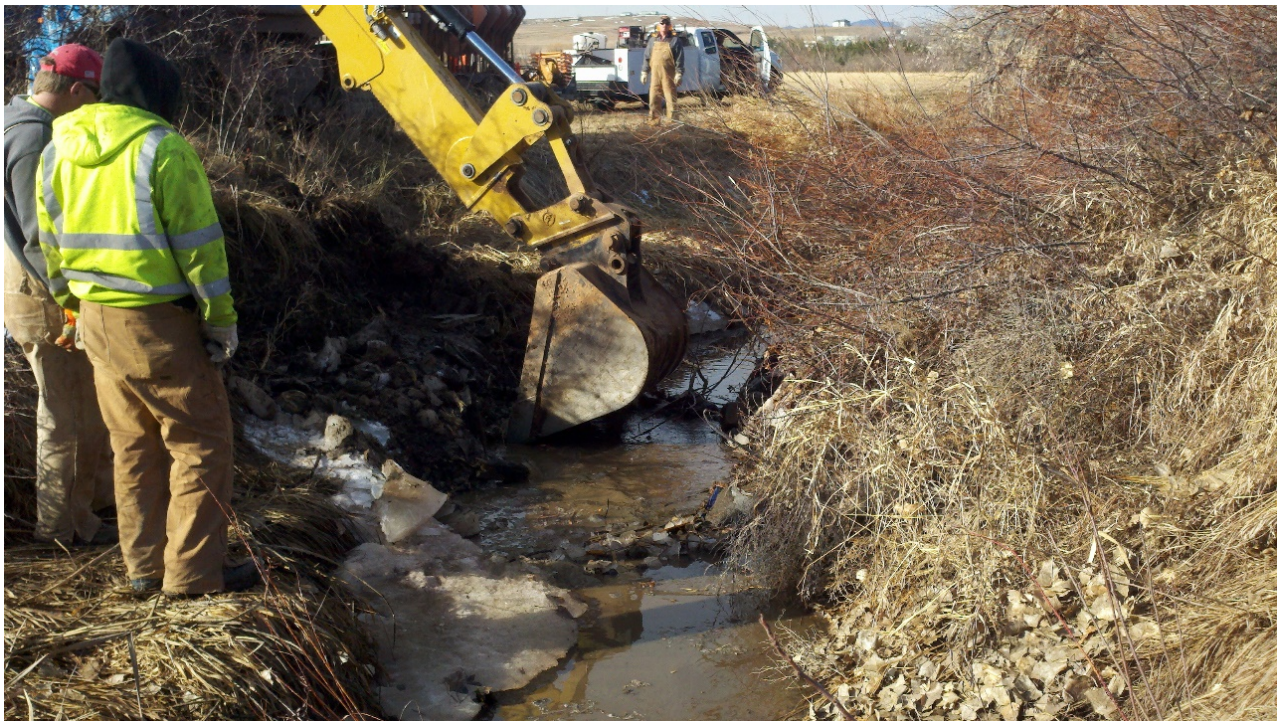
Figure 3-4. Removal of Turnout associated with Permit 2316-2. Date 3/20/2014
