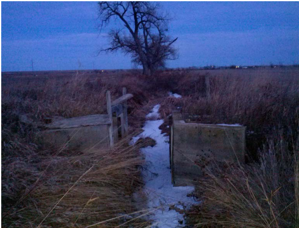
Figure 3-47. Concrete Flume/Check Structure for Turnout D Associated With Permit 2415-2 (Looking Downstream).
