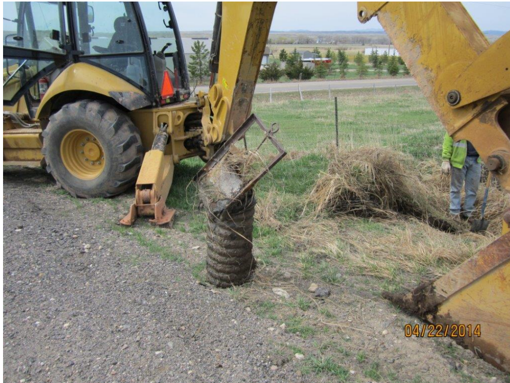
Figure 3-15. Removal of Turnout B for Permit 2399-2 Located on Murphy Ditch on Radar Road. Date 4/22/2014
