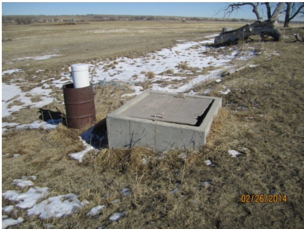
Figure 3-25. Inlet Structure, Weir Box, and Air Vent Associated With Turnout 2513-2.
