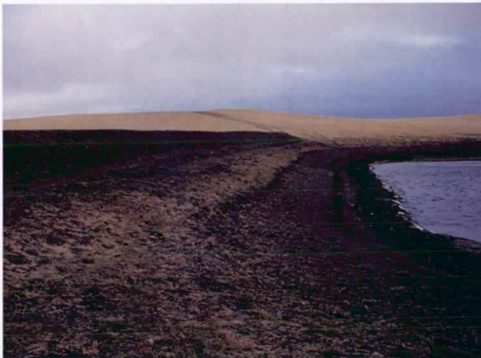
Picture of dam face (looking north)
