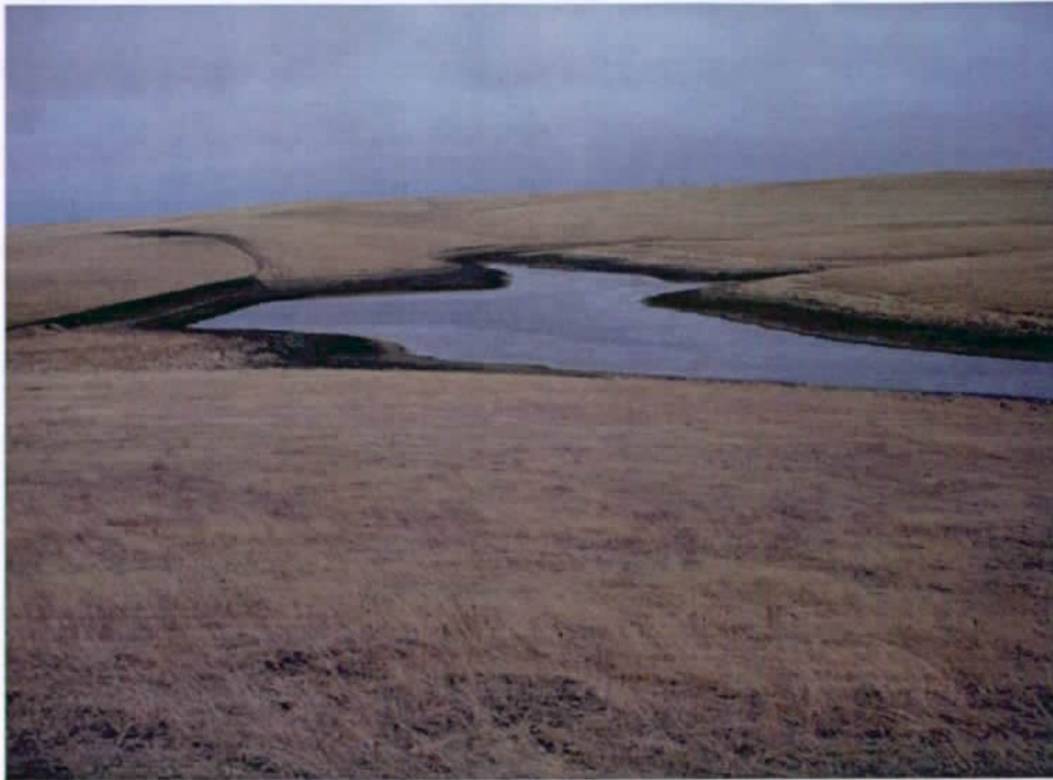
Picture of dam looking north
