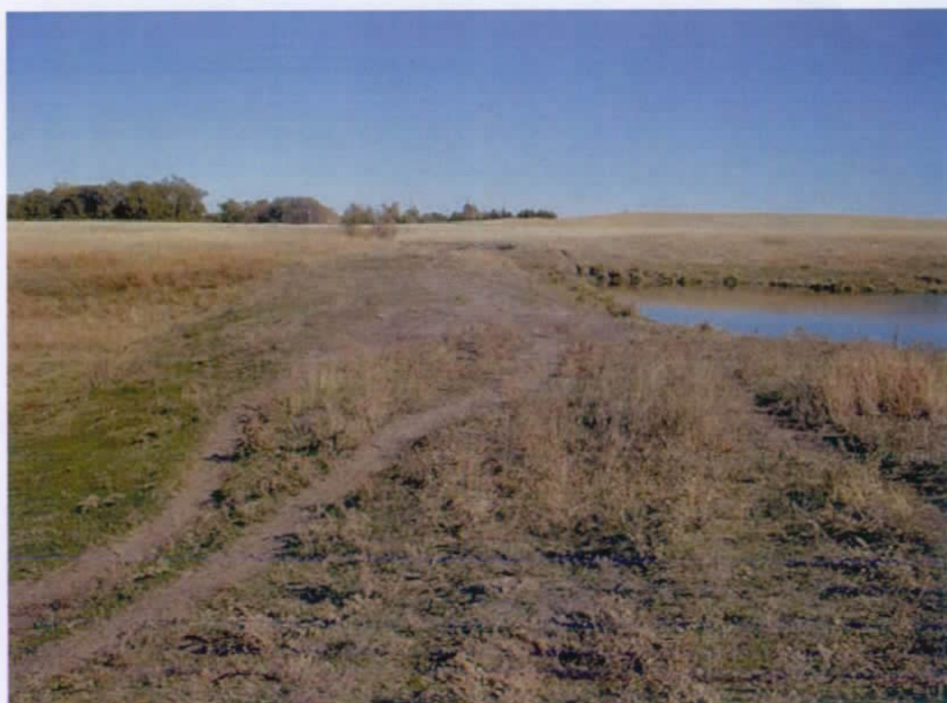
Dam # 2 (looking east)
