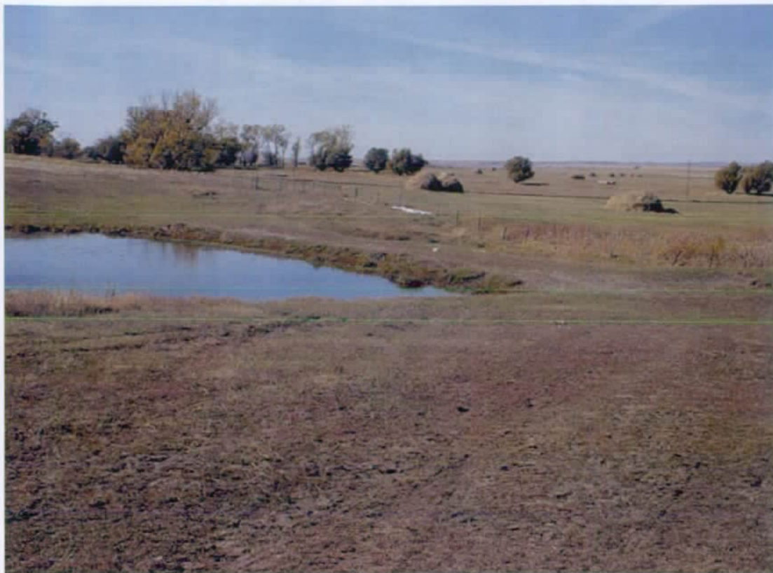
Dam No. 1 (looking west)
