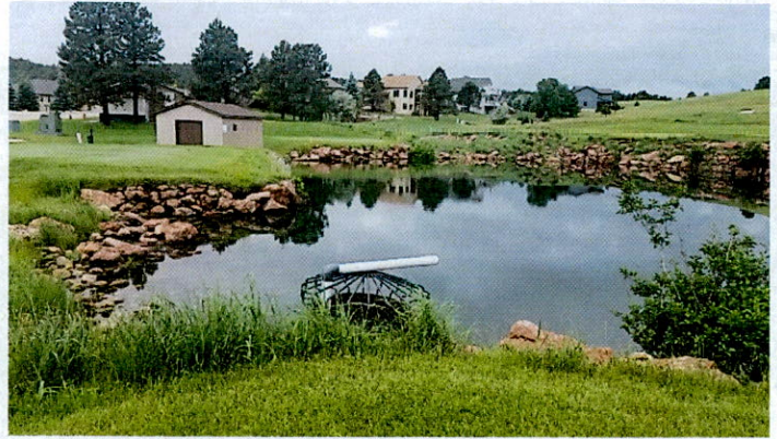
PVC supply from Dakota and Minnelusa wells discharging into storage pond. Metal trash rack and riser is overflow structure for pond. Pump house is situated at side of pond.
