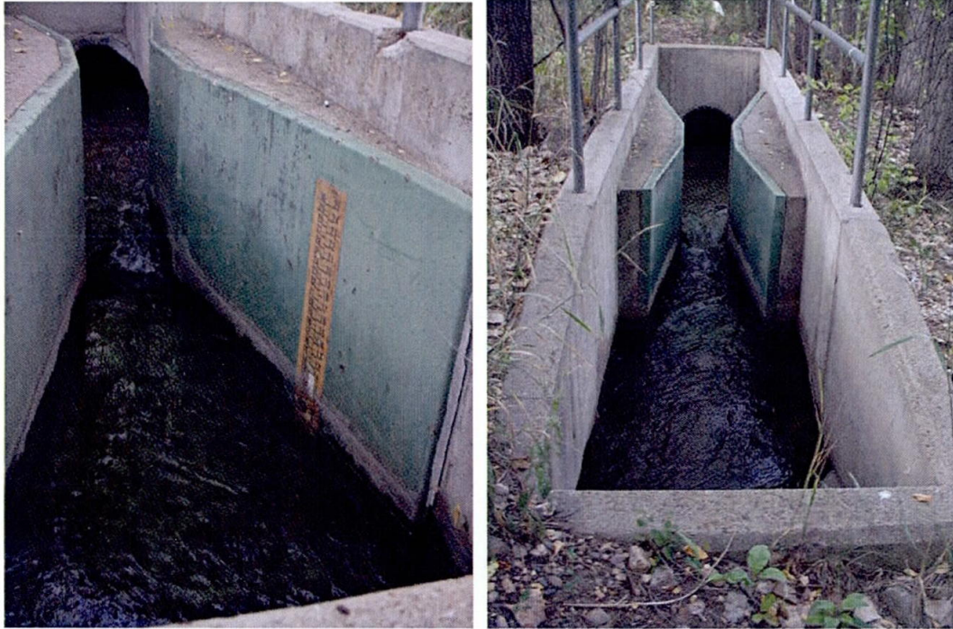
Leedy Ditch parshall flume measuring device located below Canyon Lake spillway.
