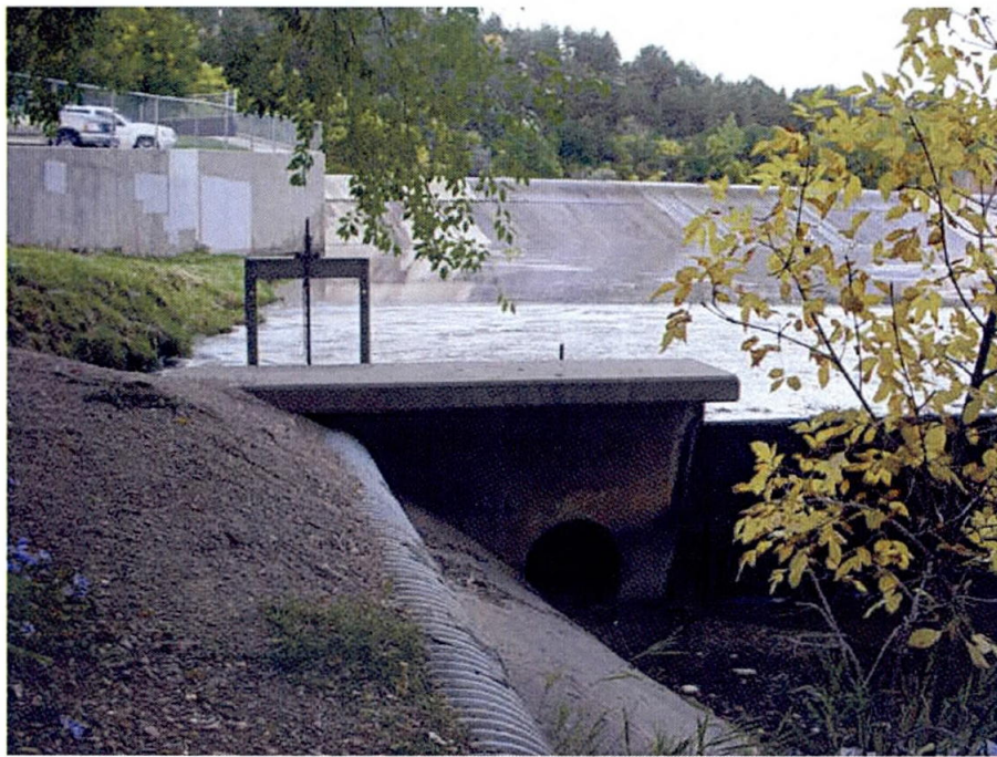
Leedy Ditch headgate located on right bank of Rapid Creek below Canyon Lake spillway.
