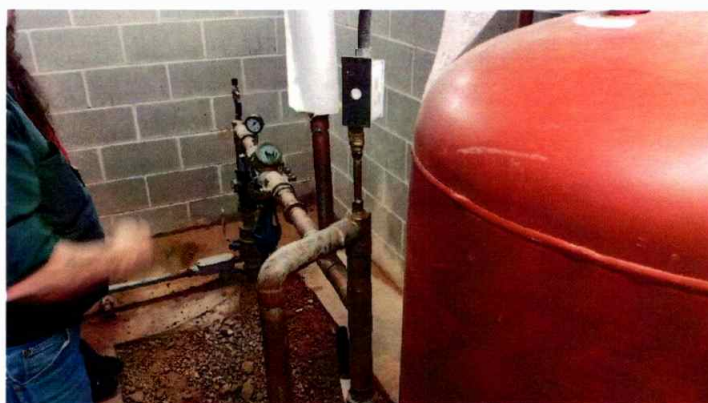
Pump house appurtenances
